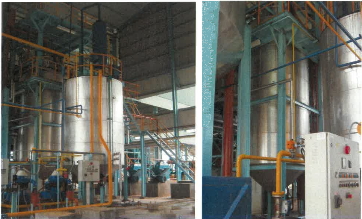
Figure 19: Pure Oil Tank And Sludge Tank
