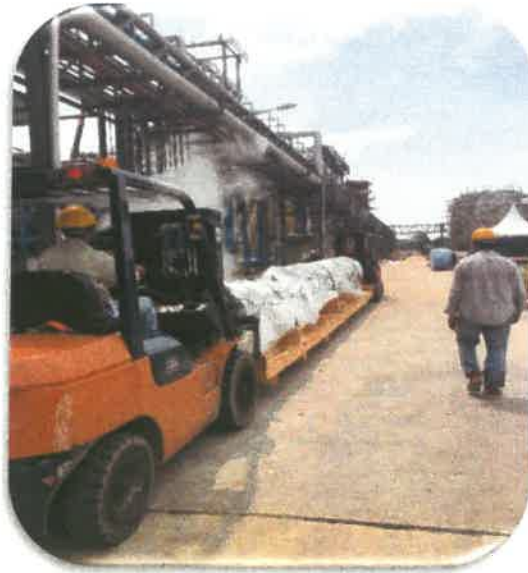
Figure 19. Worker driving forklift
