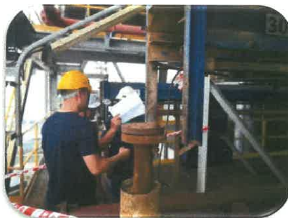
Figure 25. Discussion between engineer and supplier
