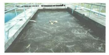
Figure 2.5 Aeration Tank of the Wastewater Treatment System at Halal Abattoir Complex
