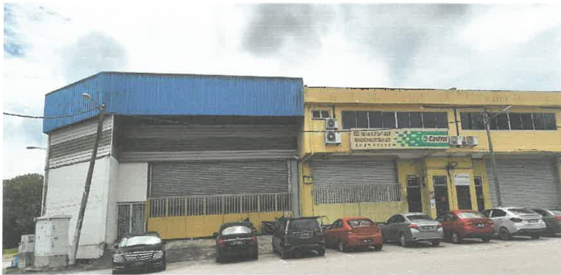
Figure 2.3: Frontal view of the office building
