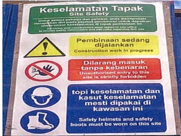
Photo 3.3.7: Site Safety Signage.
