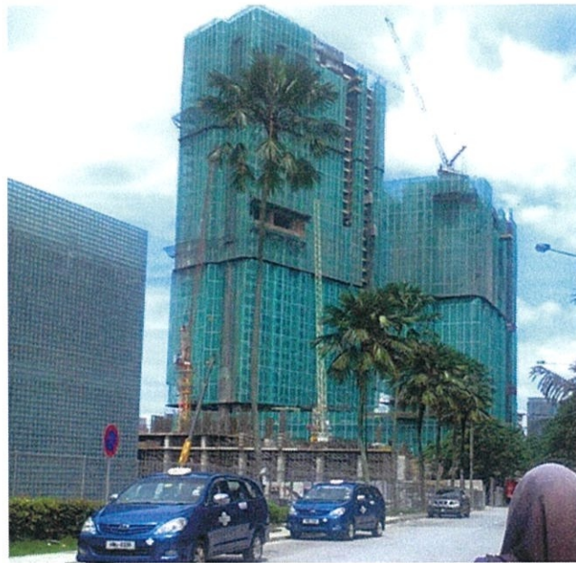
Photo 3.2 : Picture of on going project.
