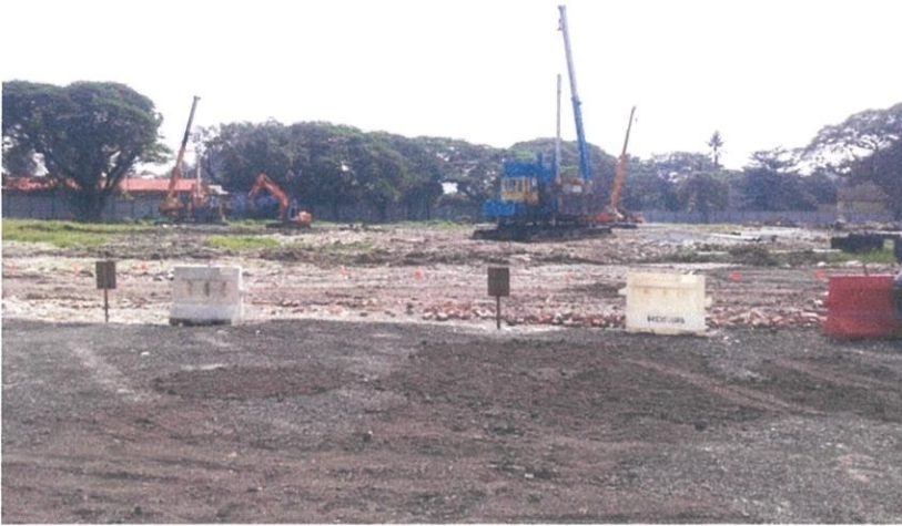
Figure 1.3.1 : Orservation at site construction ( Klinik Kesehatan Kuala Lumpur).
