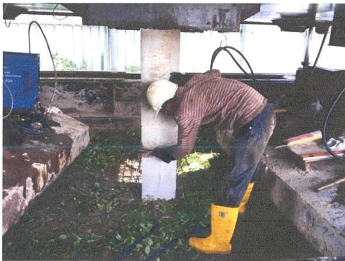
Figure 3.3.14 : The pile was being cut by the worker.
