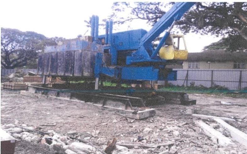
Figure 3.3.8 : Picture of Jack-in pile in construction site (Klinik Kesehatan Kuala Lumpur)
