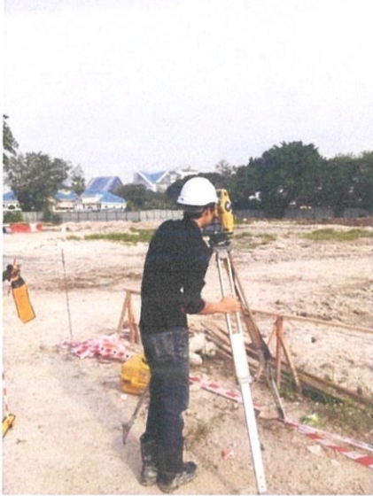
Figure 3.3.9 : surveyor doing the control point work using the tripod.
