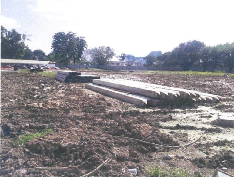
Figure 3.3.7 : Picture of pre-cast piling in site construction ( Klinik Kesehatan Kuala Lumpur)
