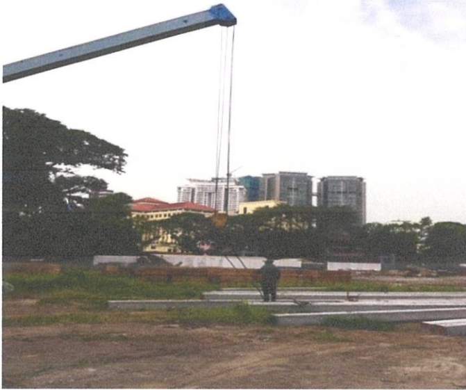
Figure 3.3.11 : The workers was clamp the pile with the crane cable.
