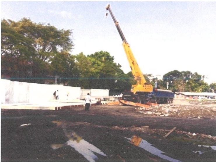
Figure 3.3.10 : The safety officer is doing a checking for the piling machine.
