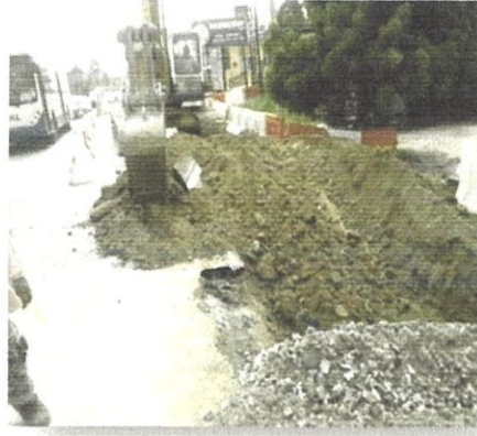
Photo 3.6 : Excavation of Pavement
