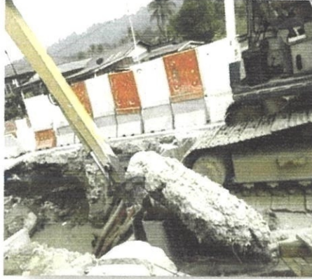
Photo 3.4 : Excavation for Piling Work
