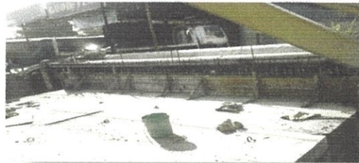
Photo 3.9 : Installation of Precast Box Culvert
