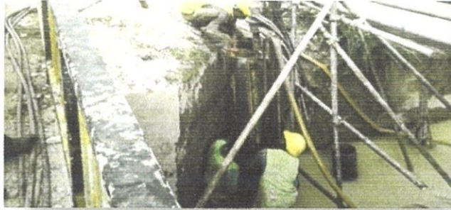
Photo 3.7 : Drilling Pile Work
