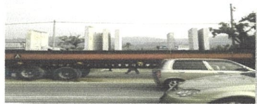
Photo 4.0 : Carry out the Precast Box Culvert
