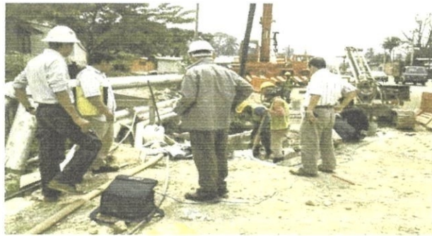
Photo 3.8 : Additional Pile Work
