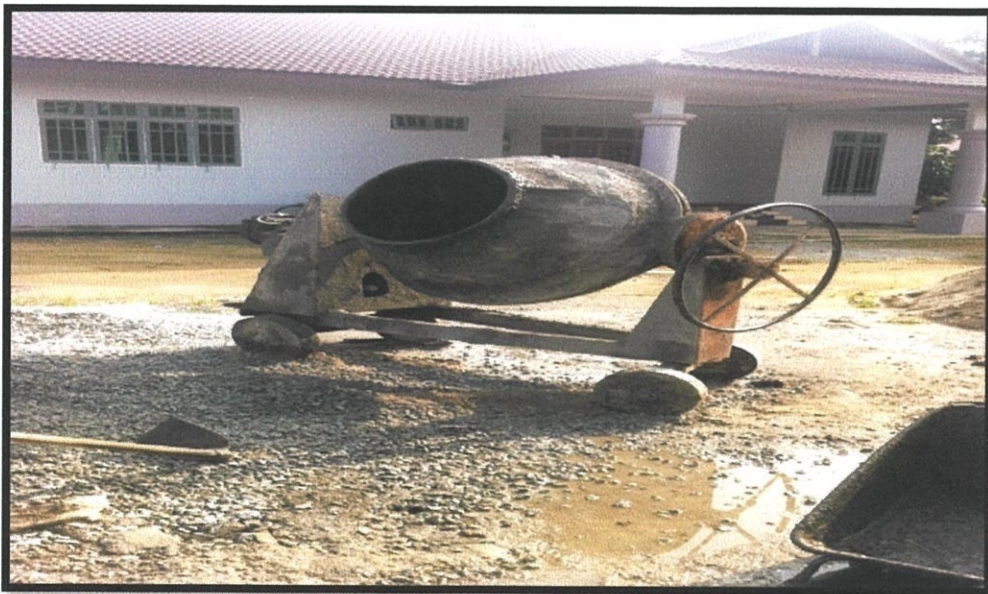
Figure 3.13: Concrete mixer used to mix the concrete at construction site.
