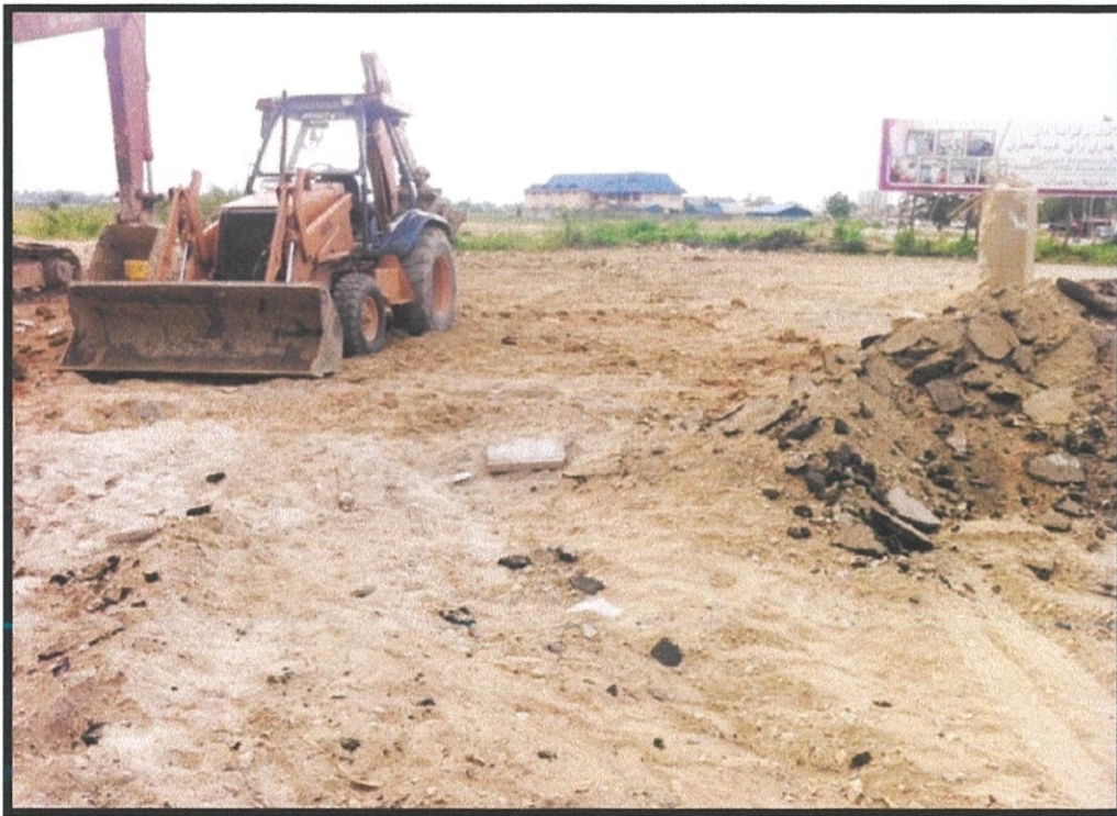
Figure 3.2: Excavator used to clear the site before construction start.
