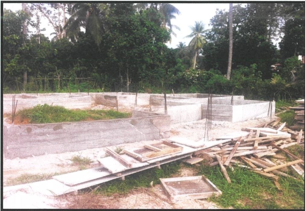
Figure 3.11: Work to remove formwork totally completed.
