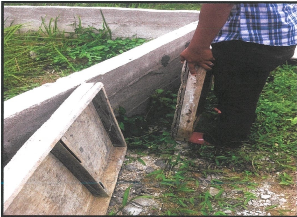
Figure 3.10: Unskill worker remove formwork after concrete totally dry.
