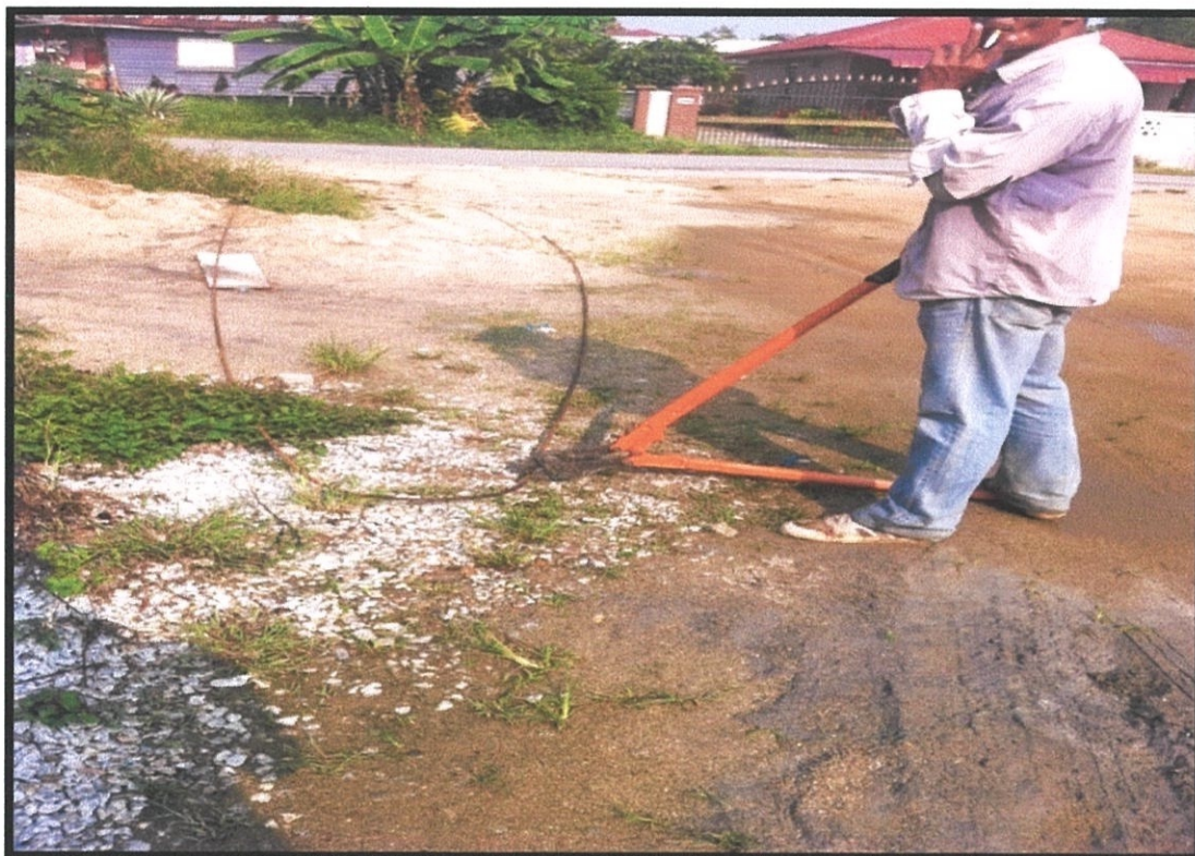
Figure 3.6: Skill worker cut the reinforcement bar by using cutter.
