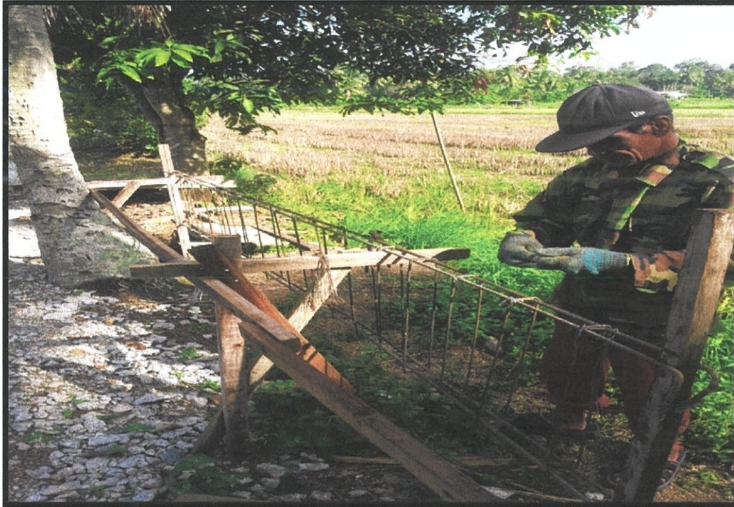
Figure 3.7: Skill worker used steel wire to tied reinforcement.
