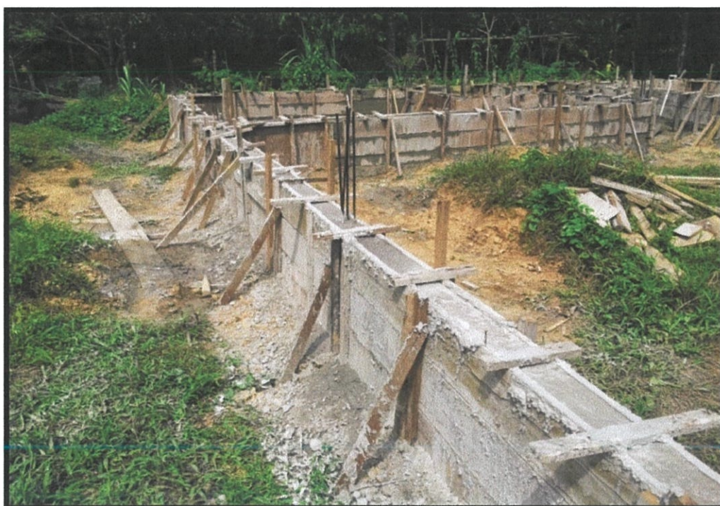
Figure 3.9: Work to infill concrete into formwork high as 3 feet.
