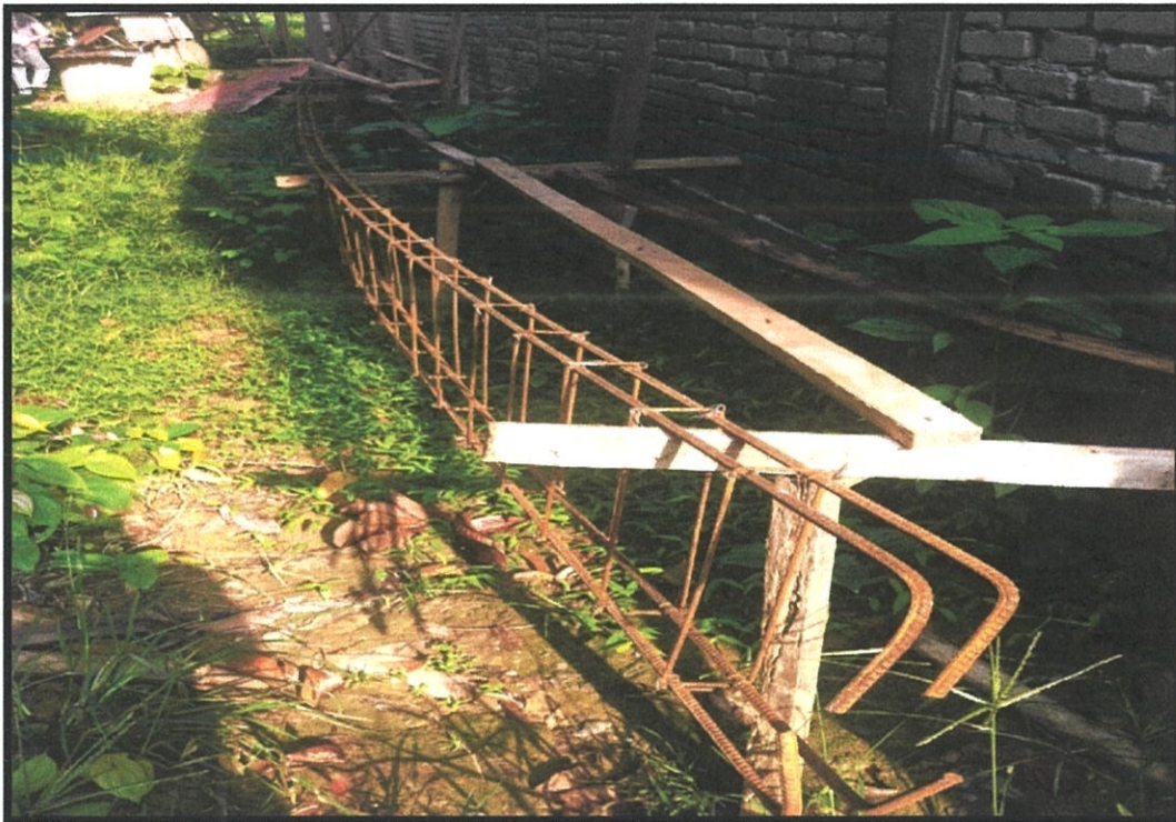
Figure 3.8: Reinforcement bar completed and ready to install.
