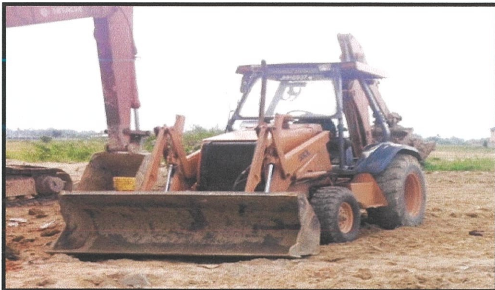
Figure 3.12: Excavator used to clear construction area.
