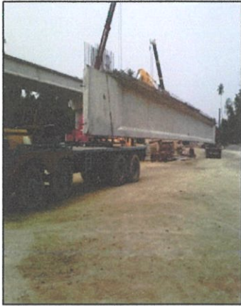
(g) Delivery T-beam by two prime mover
