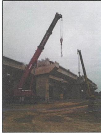
(h) Lifted T-beam on crosshead
