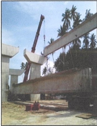
(a) Lifted T-beam by two crawler crane
