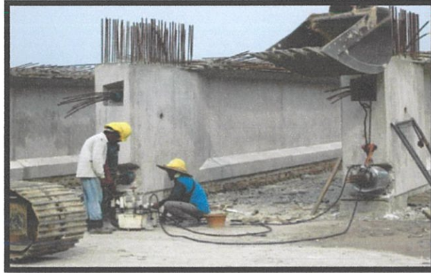
Photo 3.14 : Prestressing work for T-beam
