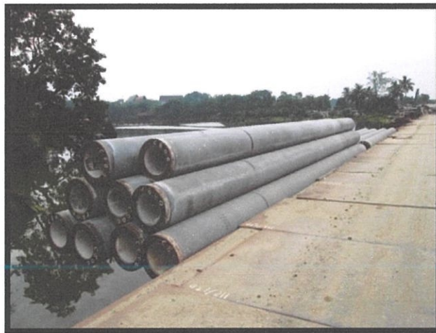
Photo 3.2: Precast Pre-stressed Spun Concrete Pile
