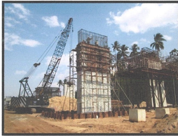
Photo 3.4: Pier Constructed
