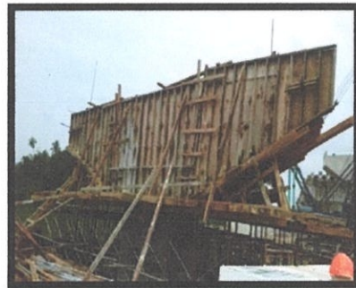
Photo 3.8: Installation of timber formwork for crosshead
