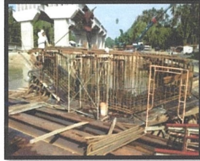
Photo 3.6: The fixing and tie in reinforcement bar.
