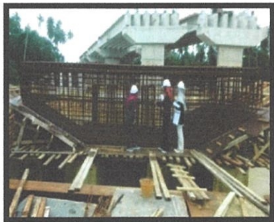
Photo 3.7: Inspection reinforcement bar for crosshead
