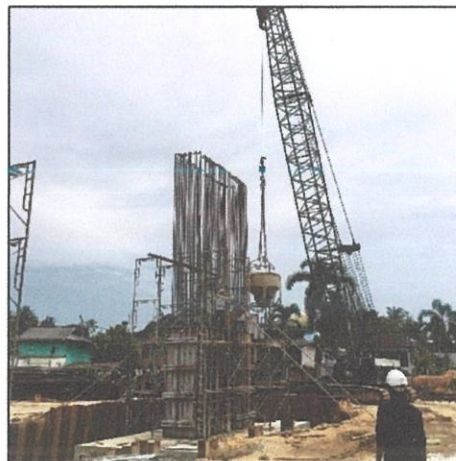
Photo 3.29: Supervisor guide the machinery during lifting concrete bucket
