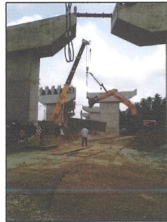
(e) Lifted T-beam by two crawler crane
