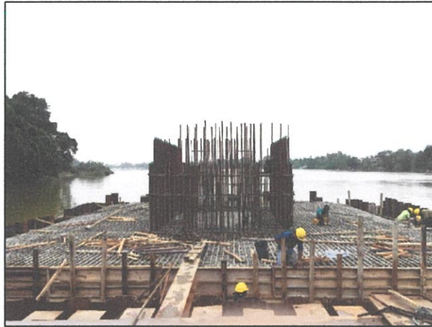
Photo 3.3: Pile Cap Reinforcement
