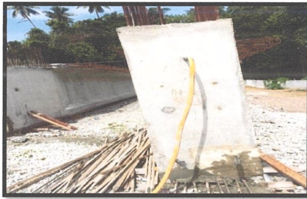
Photo 3.12 : Grouting works for T-Beam
