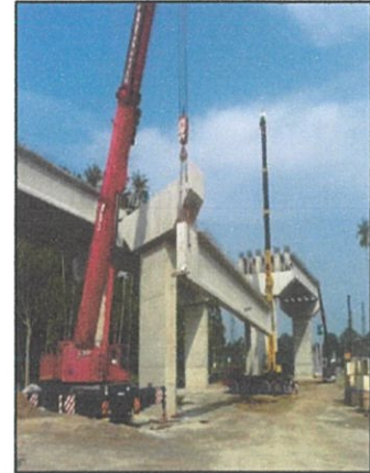
(i) Lifted T-beam by two crawler crane
