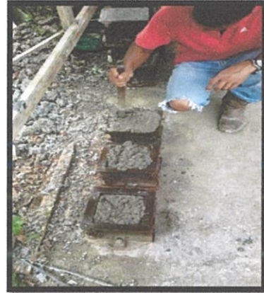
Photo 3.21: Compacting process
