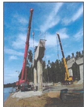
(f) Lifted T-beam by two crawler crane
