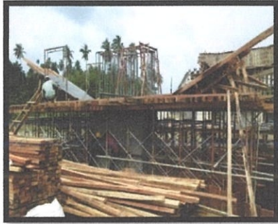
Photo 3.5: Installation of platform for crosshead
