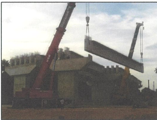
(j) Lifted T-beam by two crawler crane
