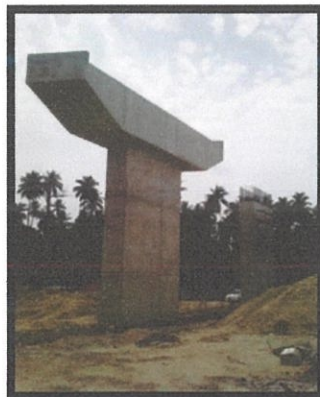
Photo 3.9: Finished Crosshead
