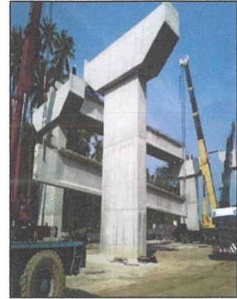
(c) Lifted T-beam by two crawler crane
