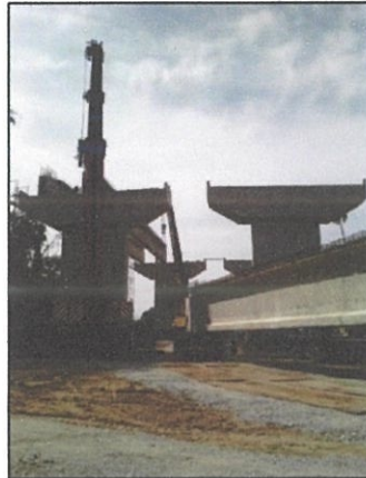
(b) Lifted T-beam by two crawler crane
