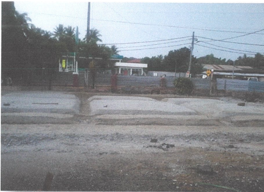
Photo 3.4 Hardcore has been compacted
