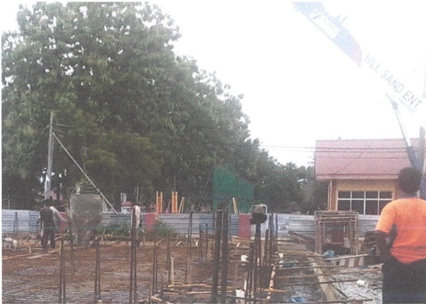
Photo 3.10 Using bucket to poured the concrete
