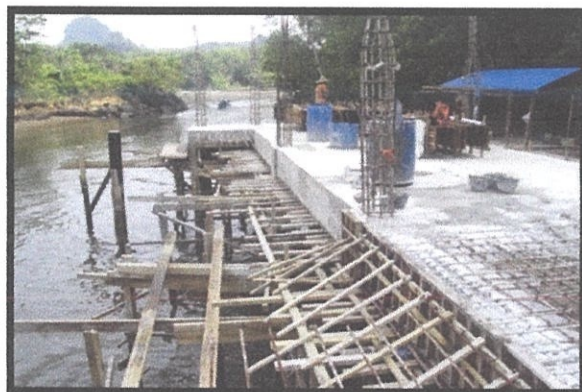
Photo 2.10 Concrete work for approach bridge
