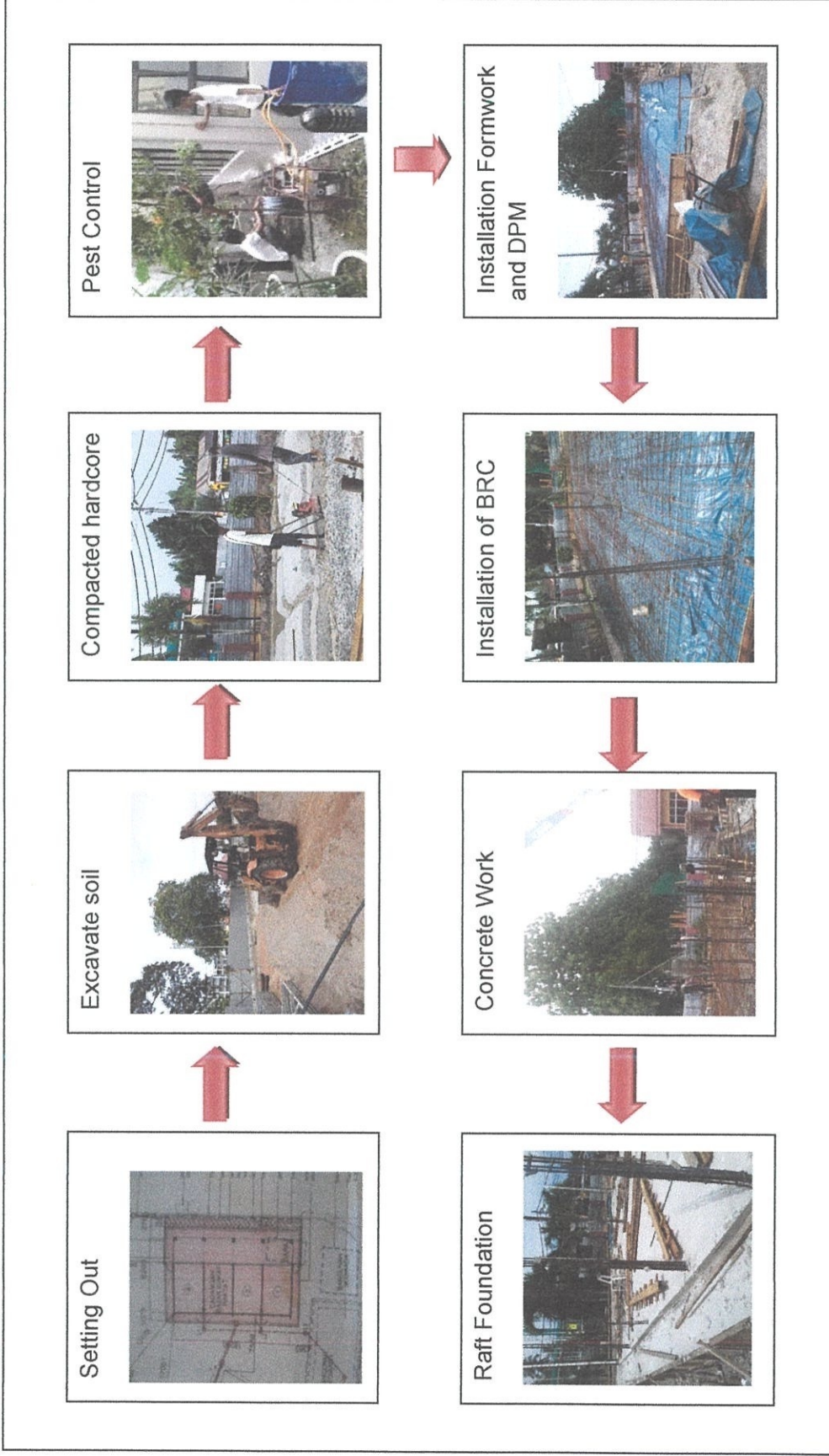
Diagram 1: Installation of raft foundation for Bazar Wakaf Rakyat
