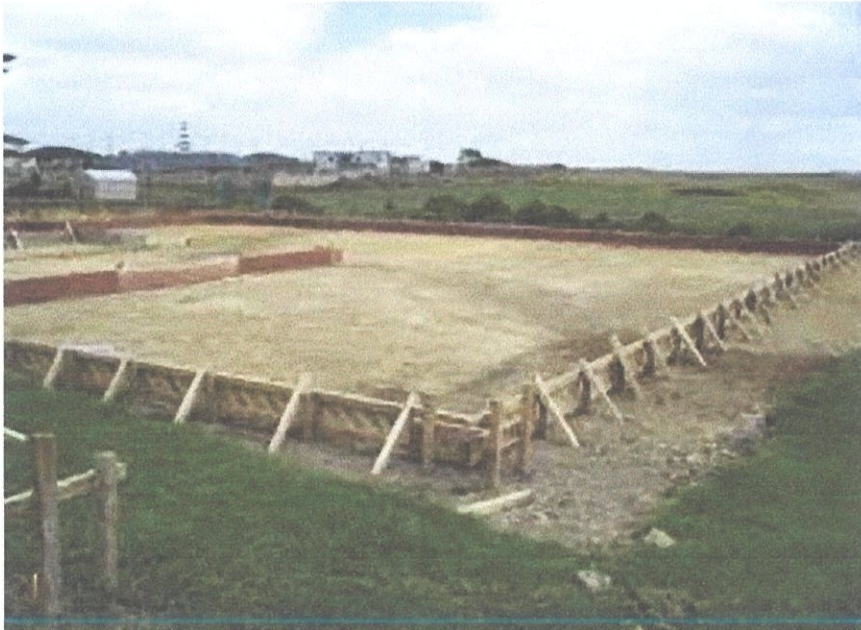
Photo 3.7 Setup the formwork
