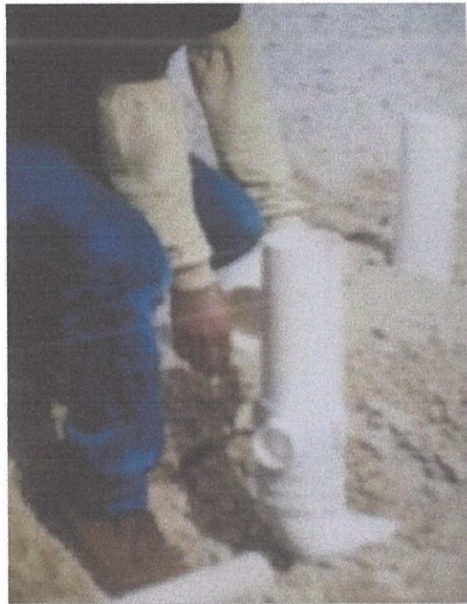
Photo 3.3 Installation of plumbing
