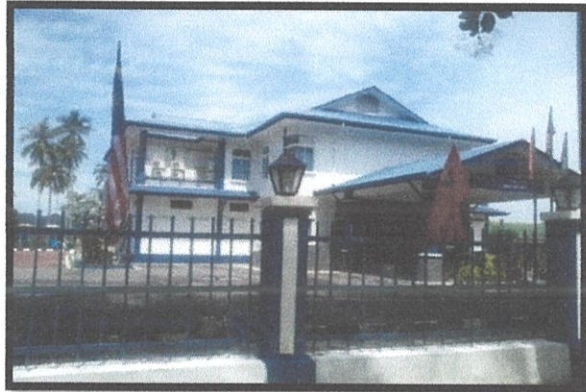
Photo 2.5 Balai Polis Ayer Hangat
