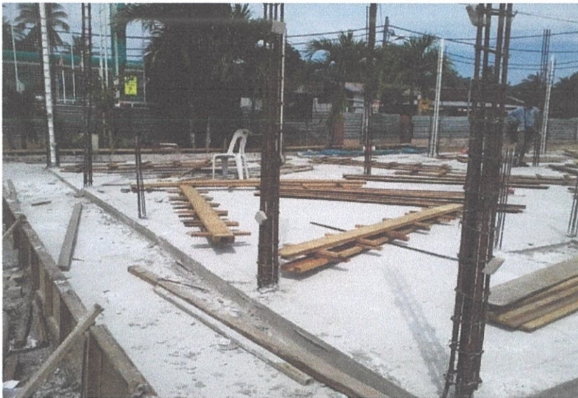
Photo 3.11 The raft foundation
