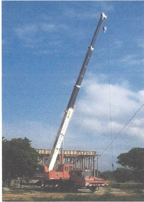
Photo 3.12 Lift up a concrete bucket use mobile crane
