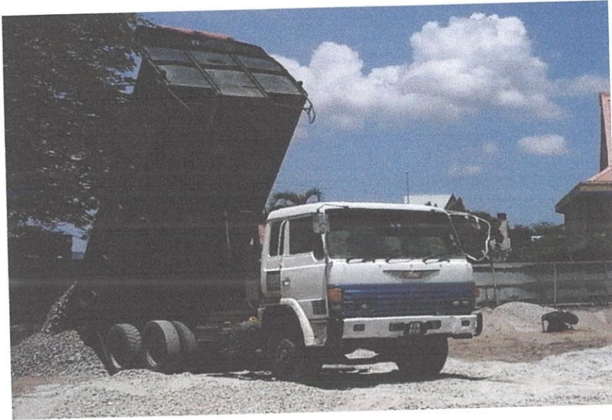
Photo 3.15 Carried sand, aggregate and hardcore to the site
