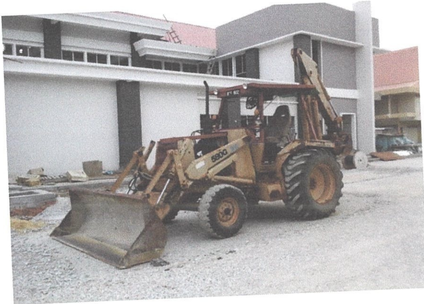
Photo 3.13 Excavator use to excavate and remove the soil
