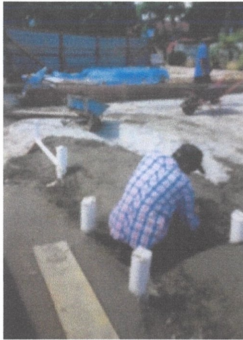
Photo 3.6 Installation of lean concrete
