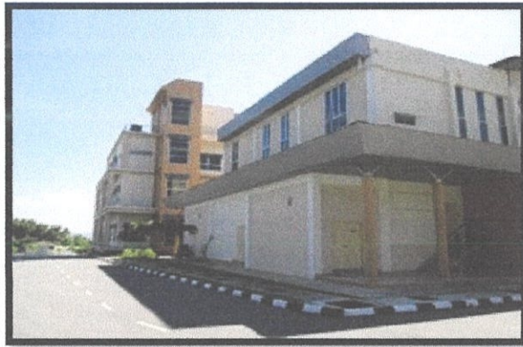
Photo 2.3 Rear elevation of Kompleks KDN Langkawi
