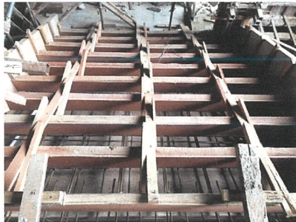
Picture 3.12 : Formwork for steps
