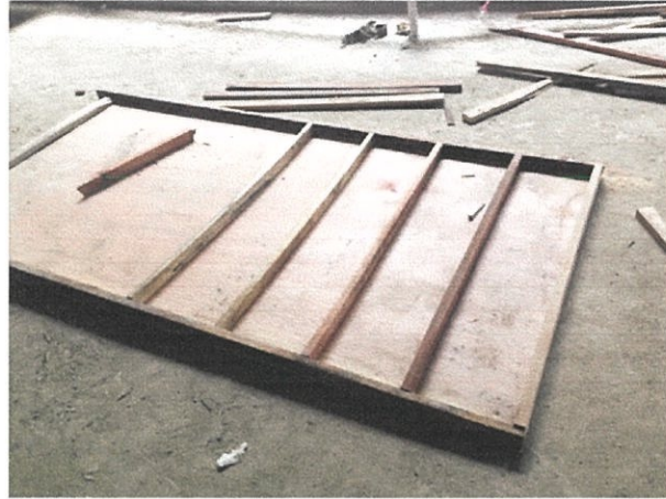
Picture 3.13: Plywood supported by a 2x3 wood
