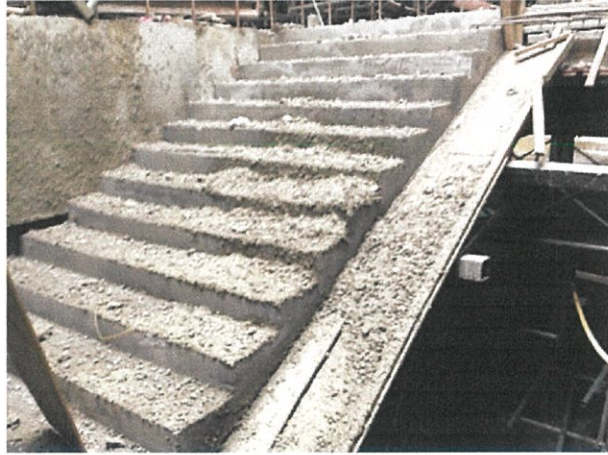
Picture 3.23: Concrete poured from upper floor
