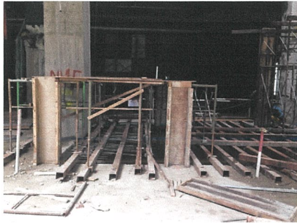
Picture 3.9 : Formwork for staircase
