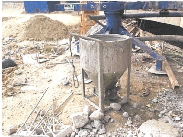
Picture 3.17 : Concrete bucket
