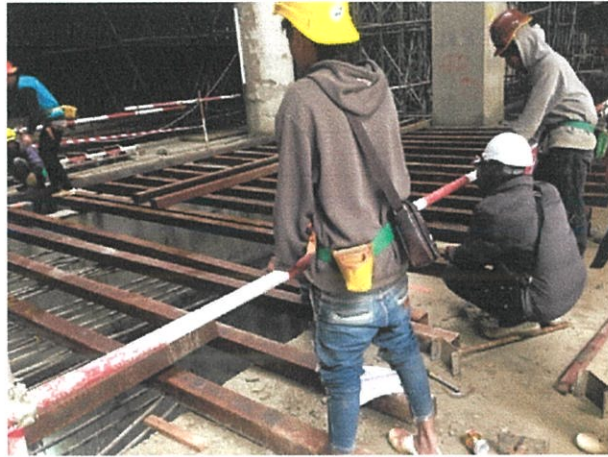
Picture 3.7 : Staging work
