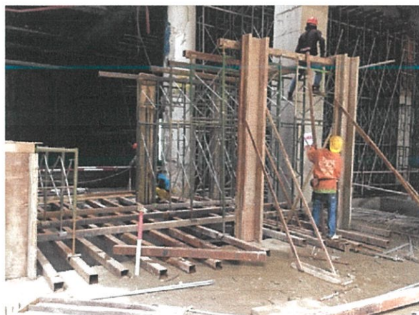
Picture 3.10 : stiffener formwork
