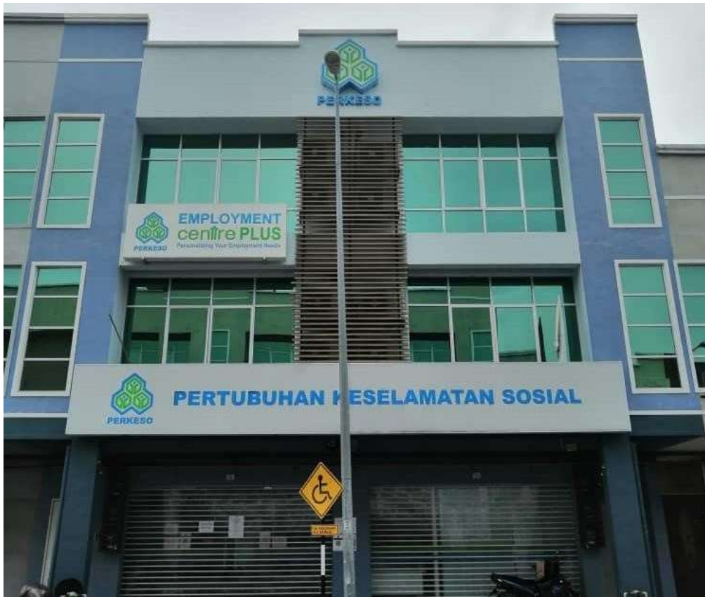
SOCSO SERI MANJUNG BUILDING
