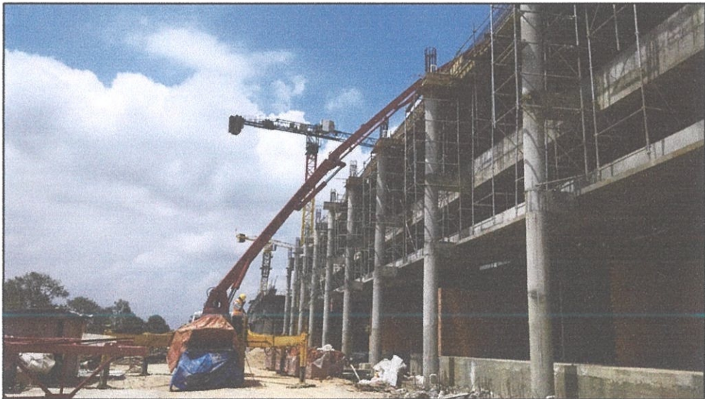
Photo 3.10 : pumping concrete to the concreting area.
