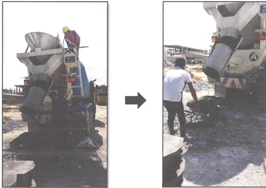
Photo 3.5 : Concrete Mixer Truck.
