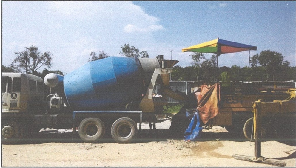
Photo 3.9 : The concrete transfer into the hopper of pump truck.
