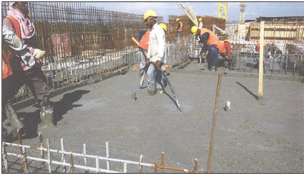
Photo 3.12 : compacting concrete.
