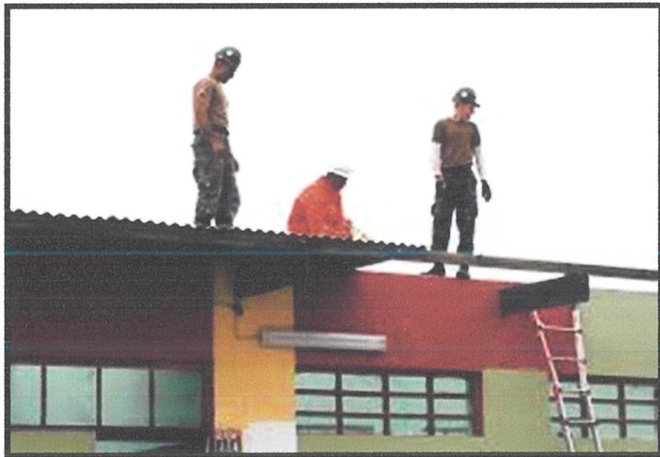
Photo 3.12 Sample of progress on maintenance
