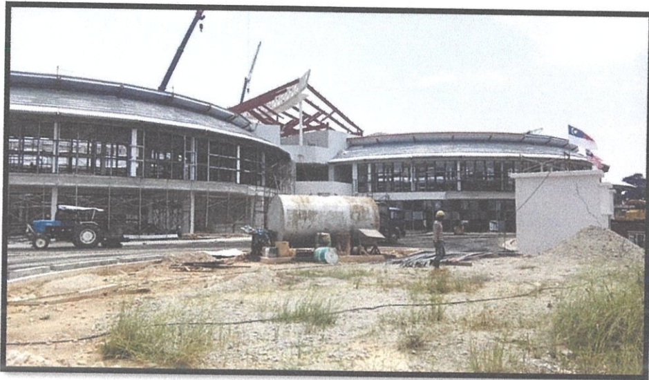
Photo 3.3: Front view of the project at 73% complete
