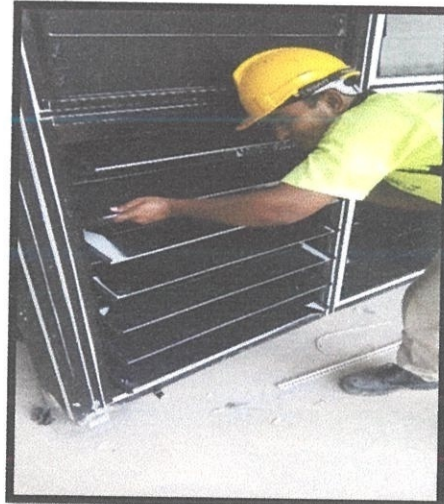
Photo 3.10: Fix aluminum blade at bottom panel before peel off protective tape
