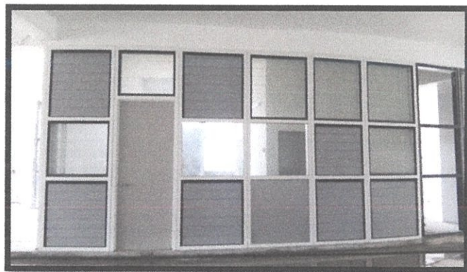
Photo 3.16: After all window installed
