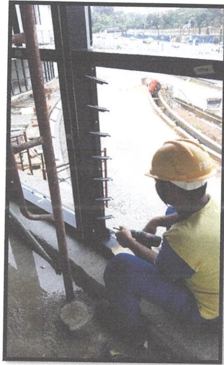
Photo 3.9: Fixing palmair adjustable
