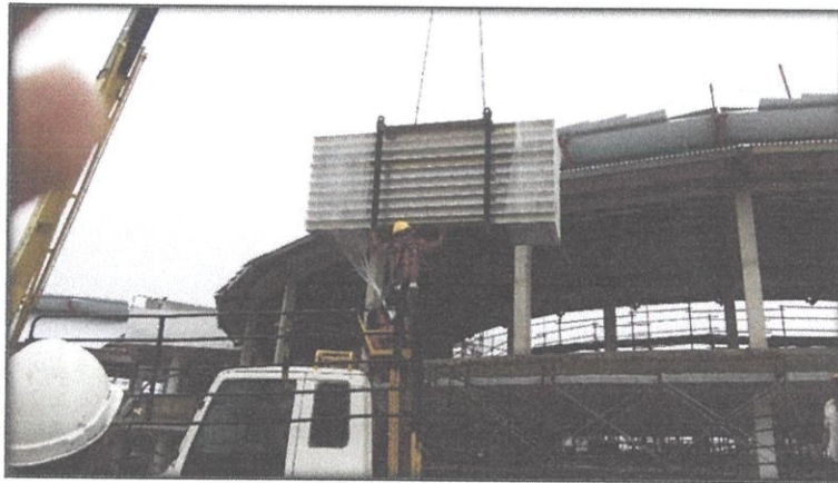
Photo 3.6: Unload window frame from lorry by car crane
