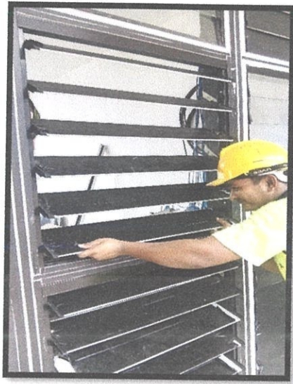
Photo 3.11: Fixing aluminum blade at middle panel before peel off protective tape
