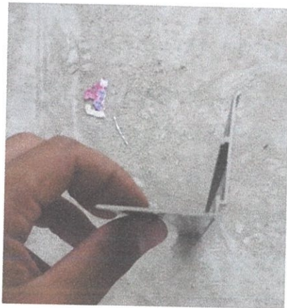
Figure 3.7: shopfront of L channel
