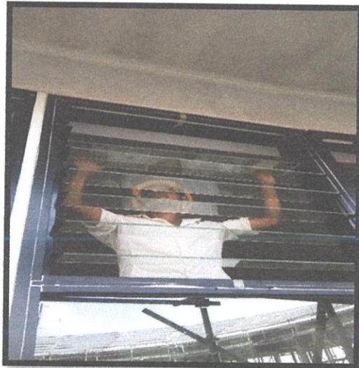
Photo 3.12: Fixing naco glass at top panel
