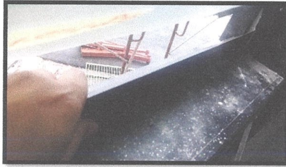
Photo 3.13: Fix L channel
