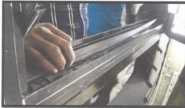
Photo 3.14: Fix weather strip
