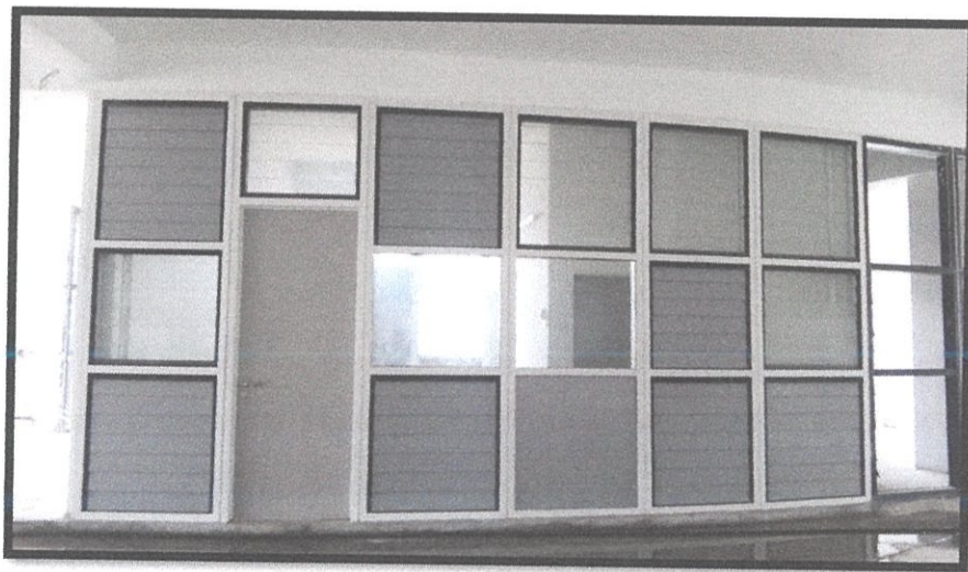
Photo 3.2: mock-up room (sample of façade window)
