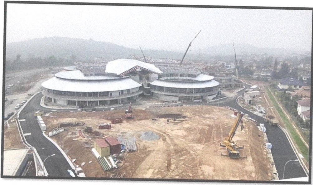
Photo 3.5: Site view from water tank elevator
