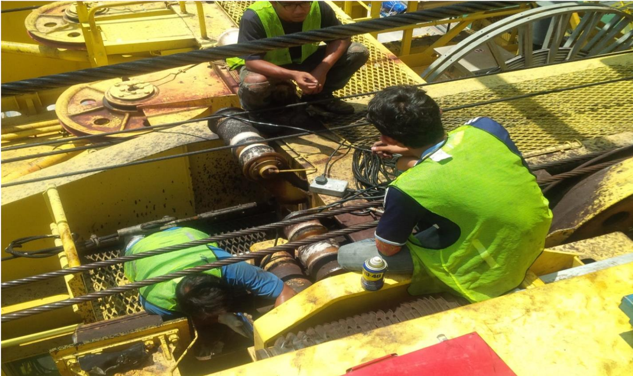
Figure 3: Repair and services Gentry Crane at Penang Port.
