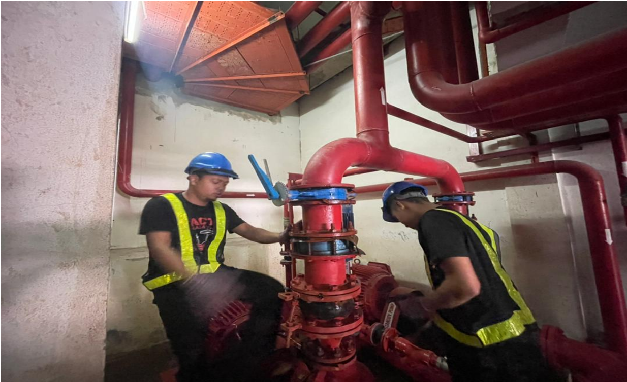
Figure 2: Repairing and services pipeline in Penang Port
