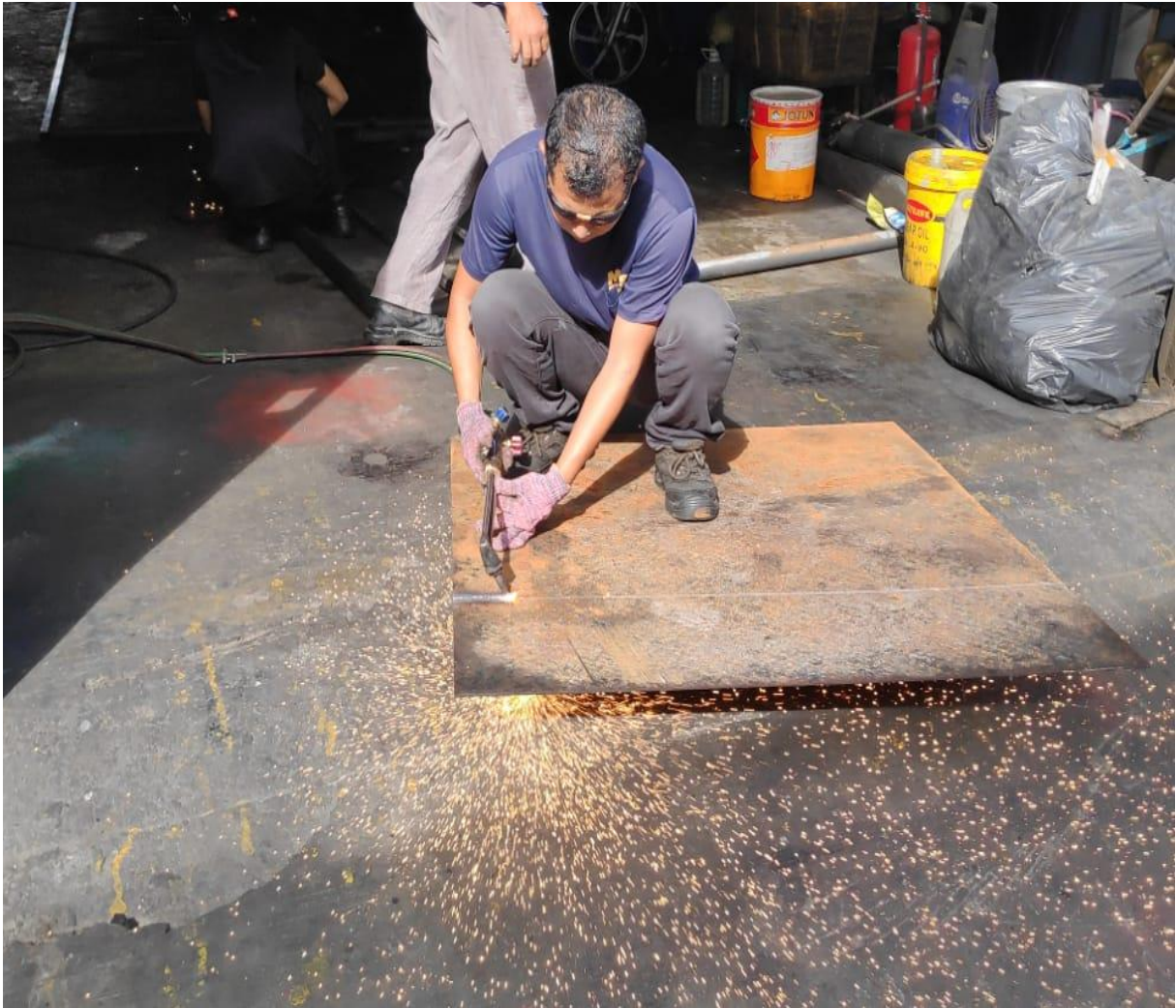
Figure 4: Cutting iron board using high flammable pressure Oxy-Acetylene
