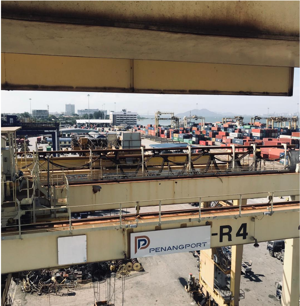
Figure 5: At the highest altitude in Penang Port
