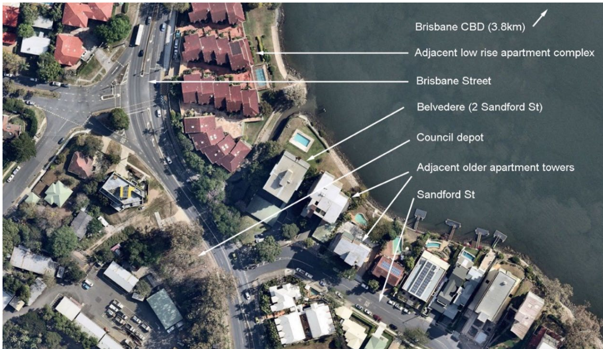
Figure 2 Area around the case study building
