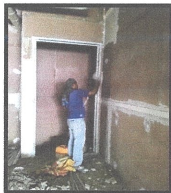
Photo 3.18: jointing process on UCO flexaboard
