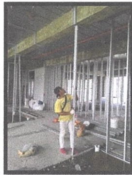
Photo 3.12: Installation of metal frame
