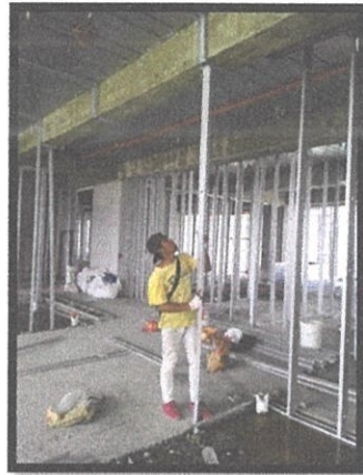
Photo 3.6: installation of wall stud
