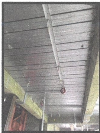
Photo 3.5: Head Track Metal Stud
