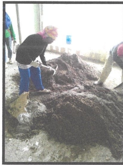
Photo 3.8: concrete mixing process
