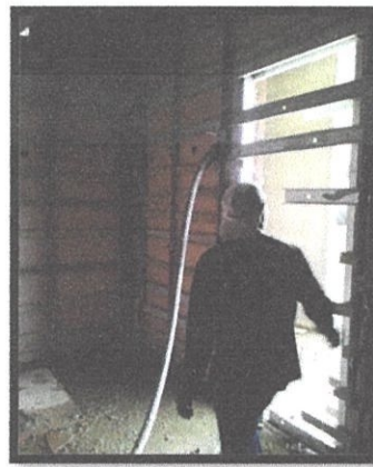
Photo 3.17: Concrete fill into UCO wall frame
