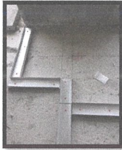
Photo 3.10: Installation of bottom stud
