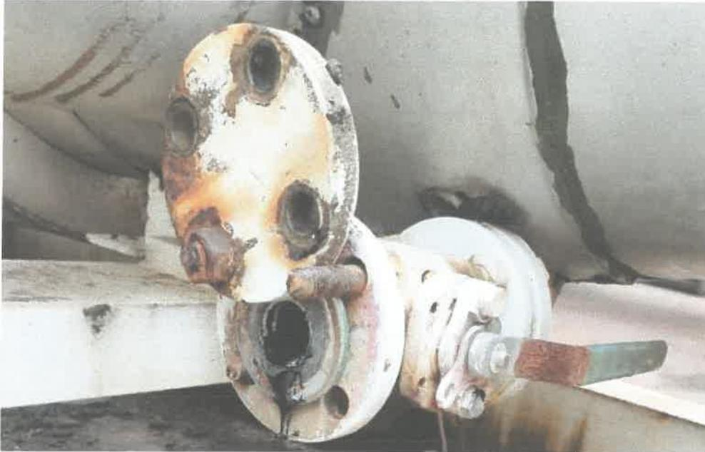
Figure 36 Liquified residue removed from the pipeline via nitrogen purging.
