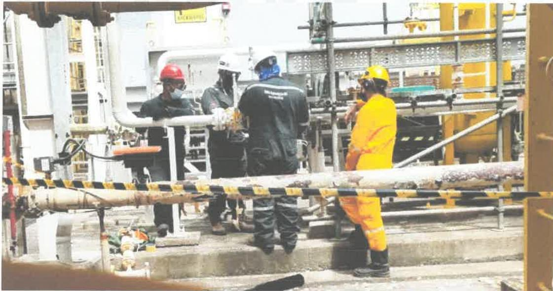
Figure 34 Contractors removing insulation on the pipeline.
