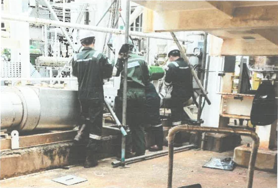
Figure 35 Operators conducting maintenance on existing supplementary firing system for H2RG pipeline.
