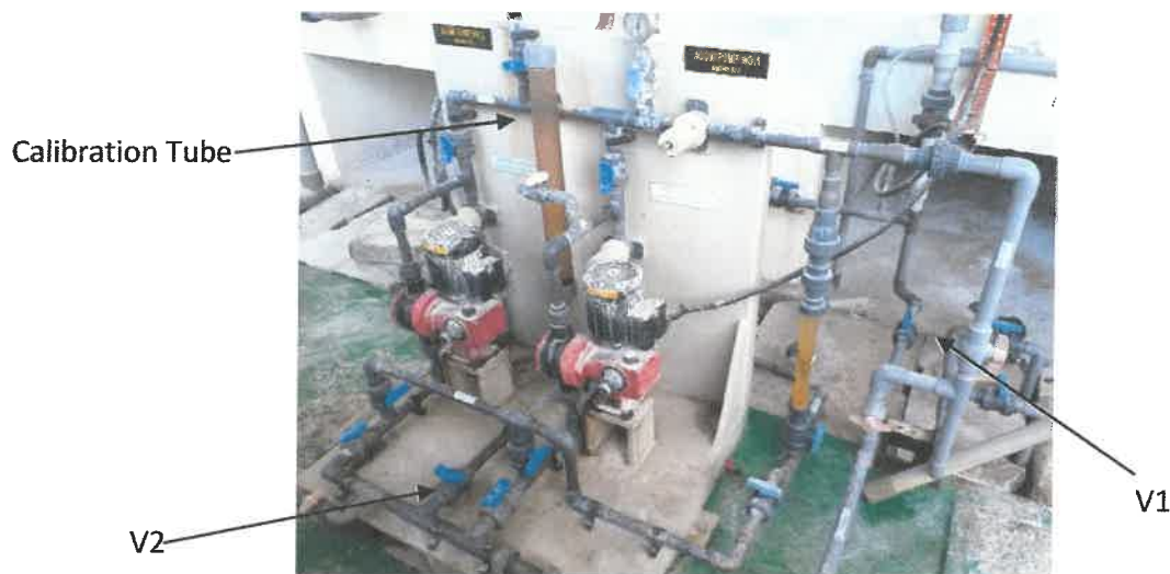
Figure 15. Chemical flowrate dosing
