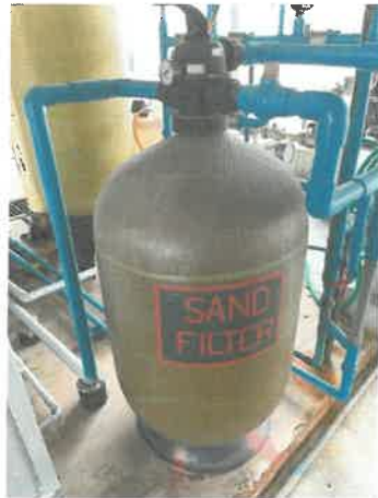
Figure 7: (a) Sand filter (b) Softener and brine tank
