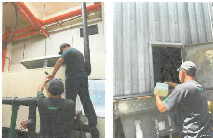
Figure 9: Chemical dosing for chiller and cooling tower
