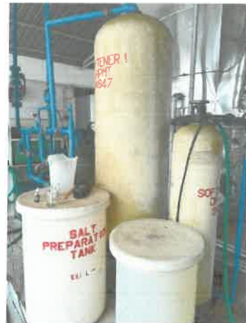
Figure 7: (a) Sand filter (b) Softener and brine tank
