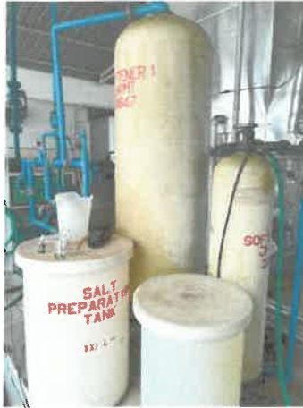
Figure 10: Resin tank and brine tank
