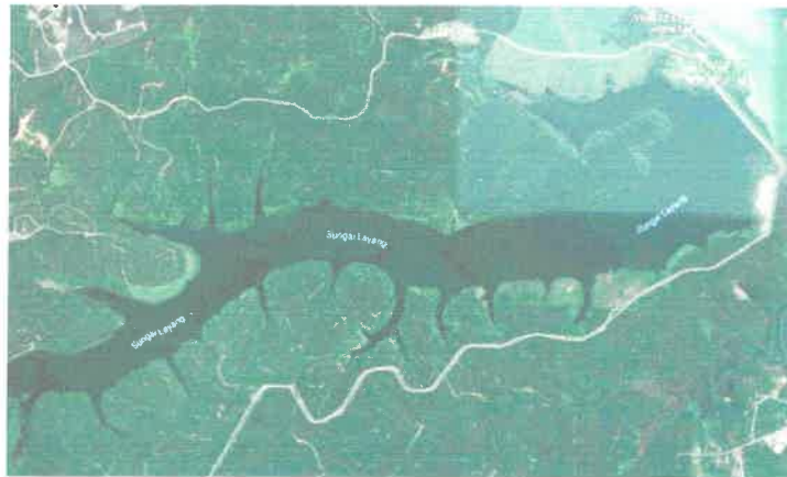
Figure 4: Picture of Lower Layang Dam
