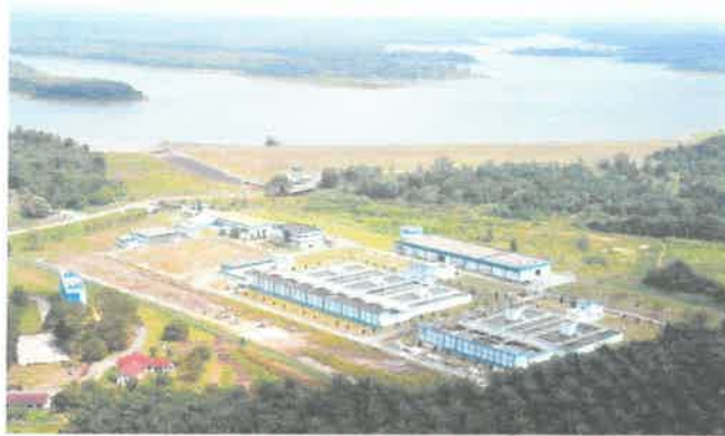
Figure 2: Water Treatment Plant Sultan Iskandar overview
