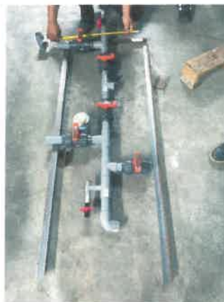
Figure 21. Bracket measurement for the piping.
