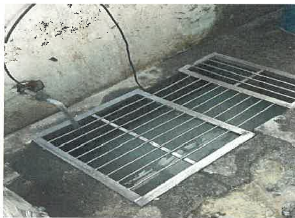
Figure 13. Raw Effluent from inside the drain
