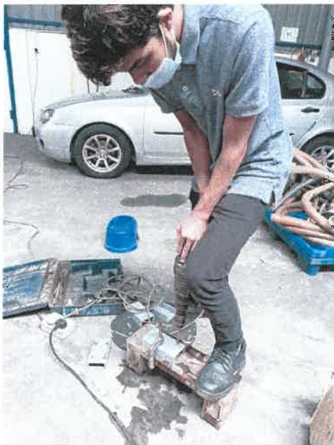
Figure 26: Drilling for Kohoku's project
