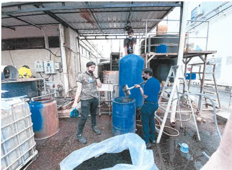
Figure 20: Servicing the activated carbon filter (ACF)
