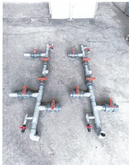
Figure 27: Face piping for Kohoku's project
