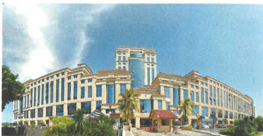
FIGURE 1: LOCATION OF ENVOSHA SDN BHD (CENTREPOINT BUSINESS PARK)
