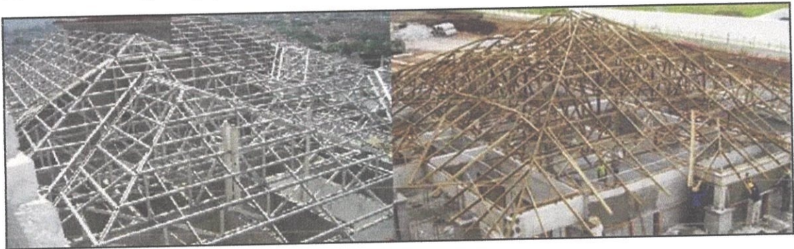
Photo 3.1 : The usages of lightweight steel and timbers as the roof truss.
