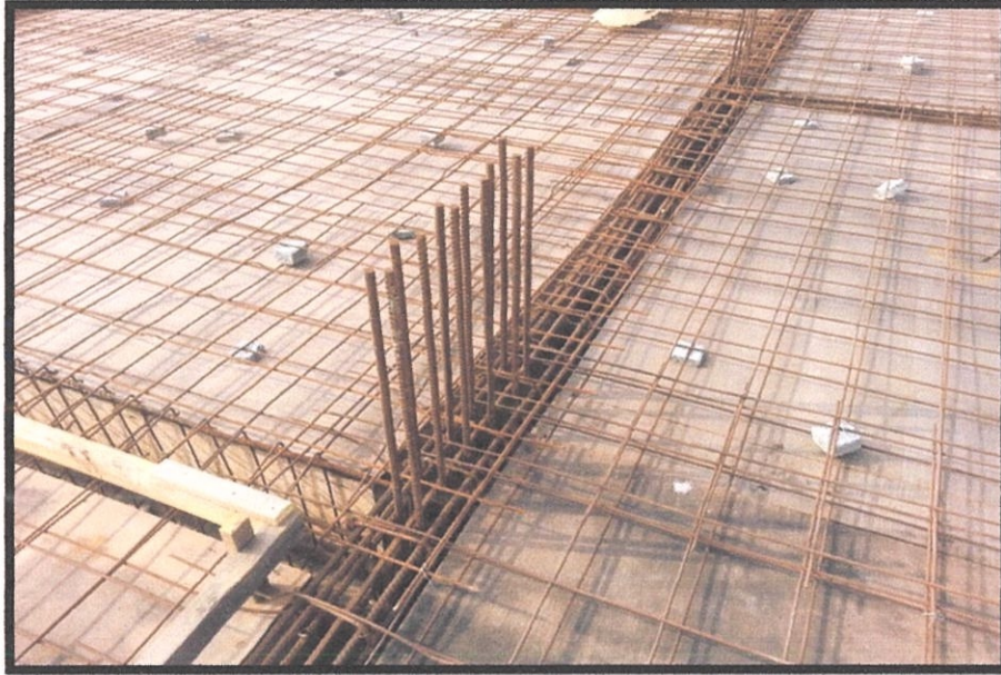
Photo 3.9 The cube between BRC and formwork called spacer
