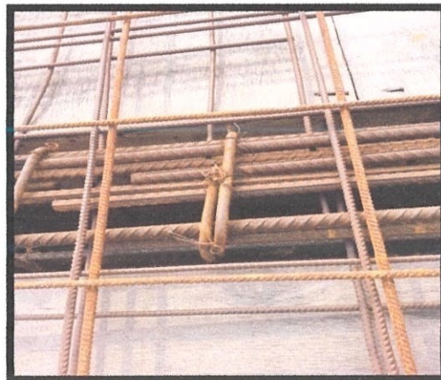
Photo 3.16 The reinforcement bar that has been bend into shape
