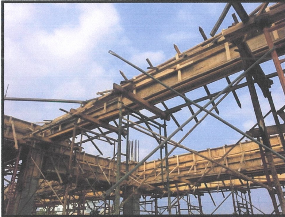
Photo 3.2 The complete formwork for 1 st floor beam
