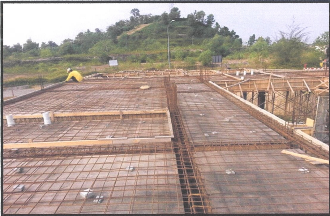
Photo 3.8 Finished result of slab reinforcement installation
