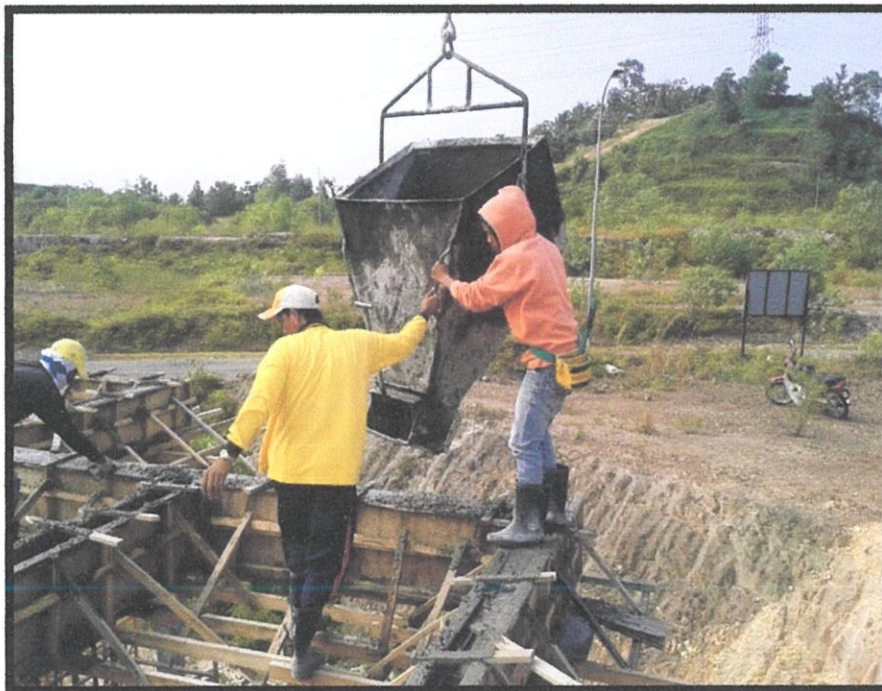
Photo 3.10 Concreting work for the beam
