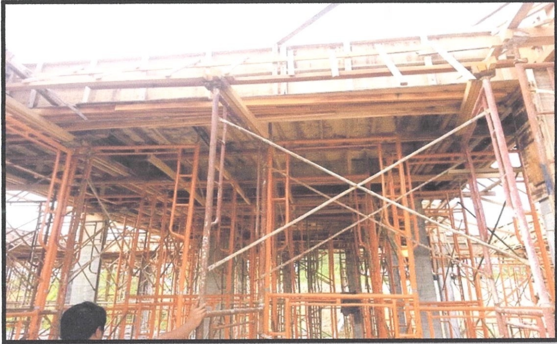
Photo 3.7 The situation on site from below after formwork installation
