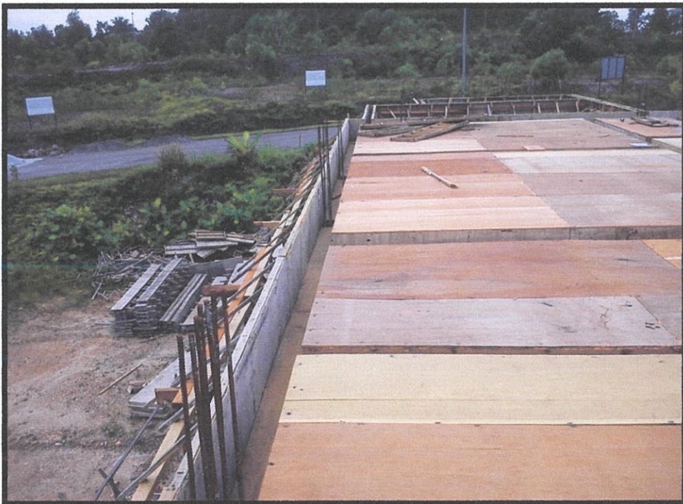
Photo 3.5 The result of slab's formwork after being installed
