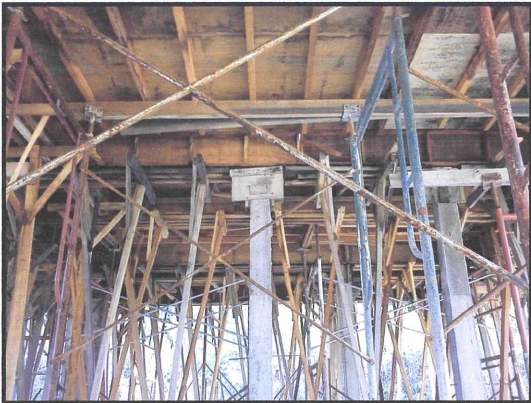
Photo 3.6 The slab's formwork supported from below
