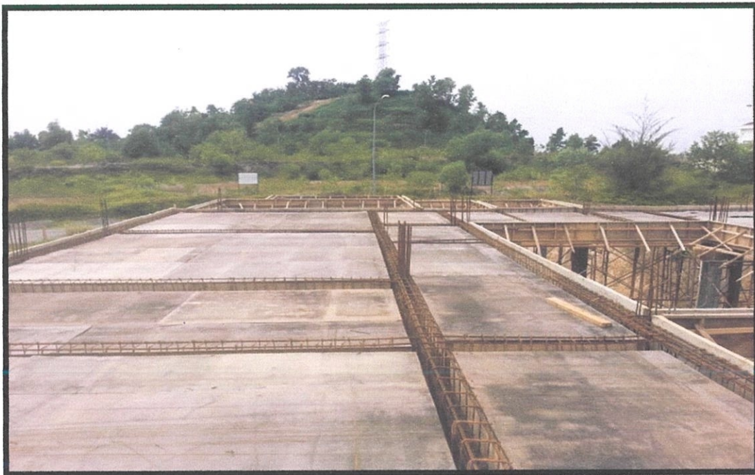
Photo 3.4 The reinforcement installation for beam is completed
