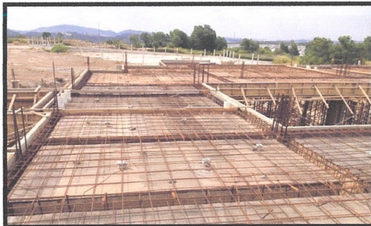
Photo 3.18 BRC that has been installed to formwork
