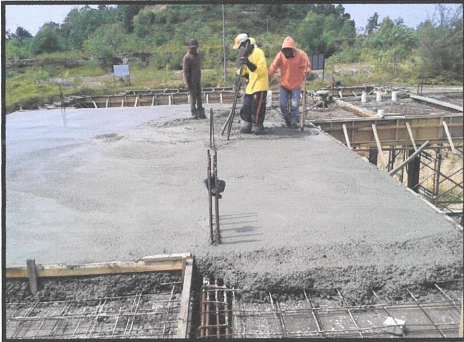
Photo 3.19 Concrete that has been poured on the slab
