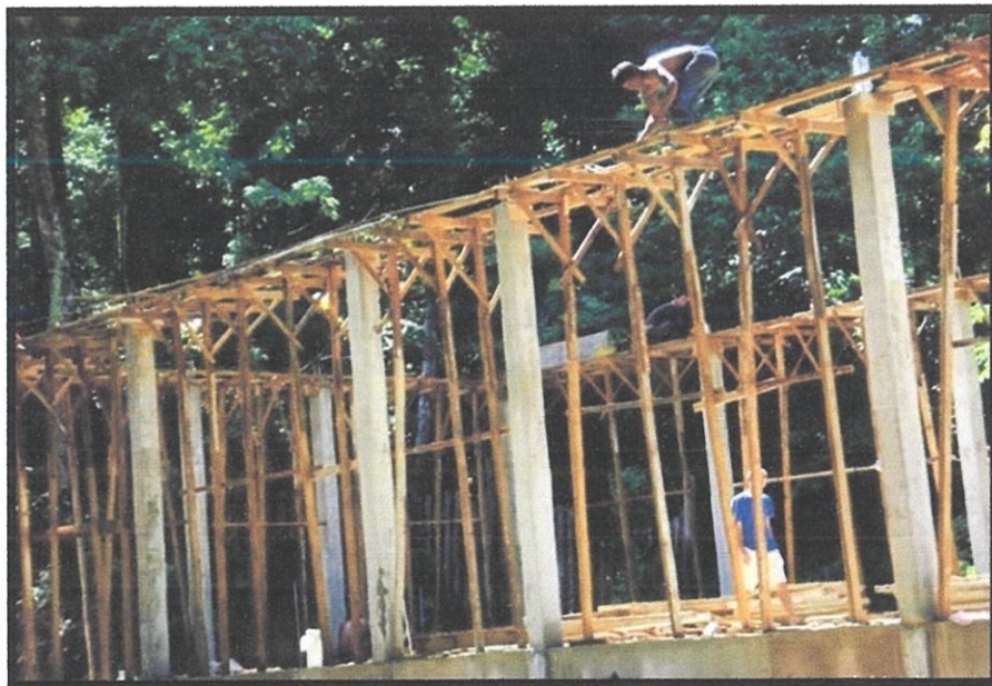
Photo 3.1 The installation of formwork for 1 st floor beam
