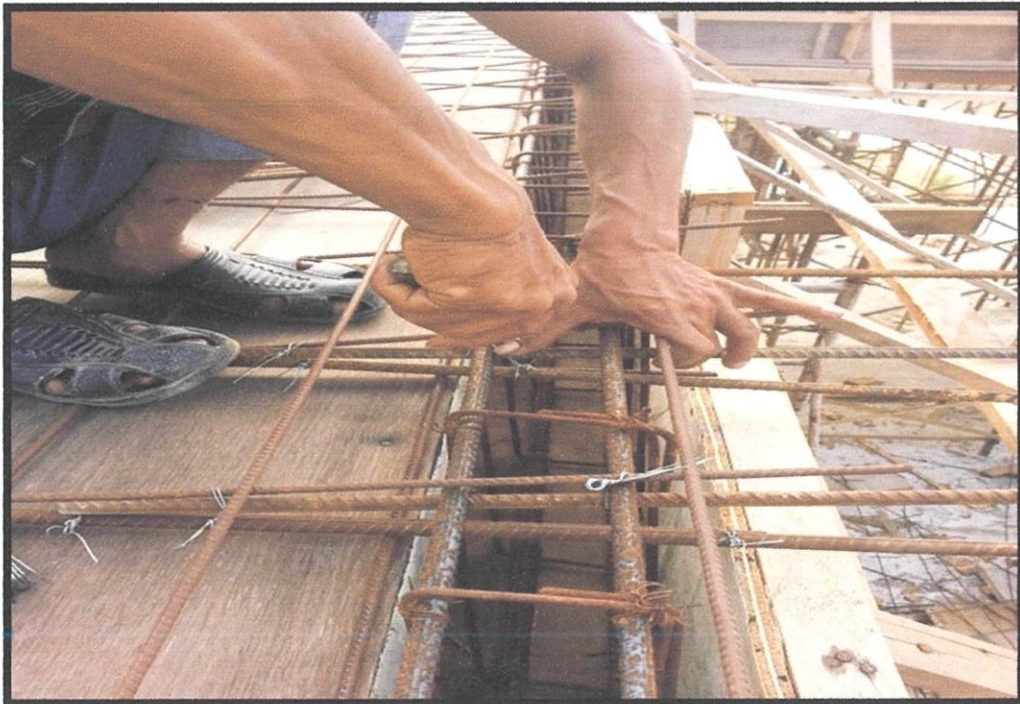
Photo 3.3 The process of tying the reinforcement bar
