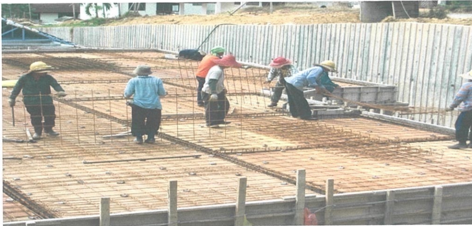
Photo 3.10 : Reinforcement bar installation to the roof slab of lockup.
