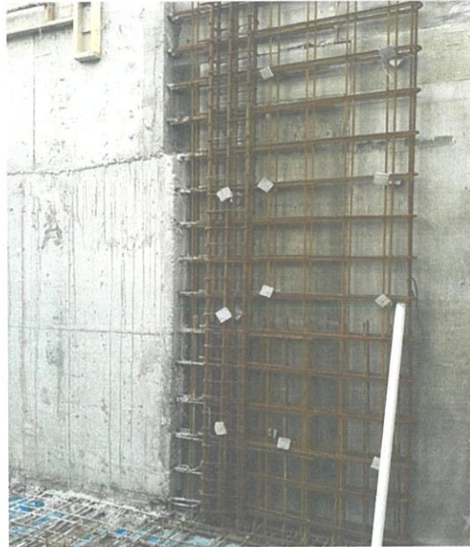
Photo 3.5 : installation of rebar at wall and floor of lockup.
