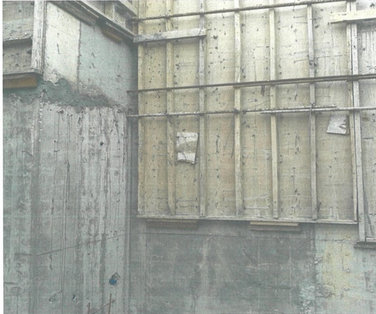
Photo 3.6 : Installation of formwork before concreting work is carry out.
