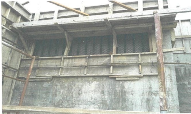
Photo 3.7 : concreting work process to wall of lockup done.
