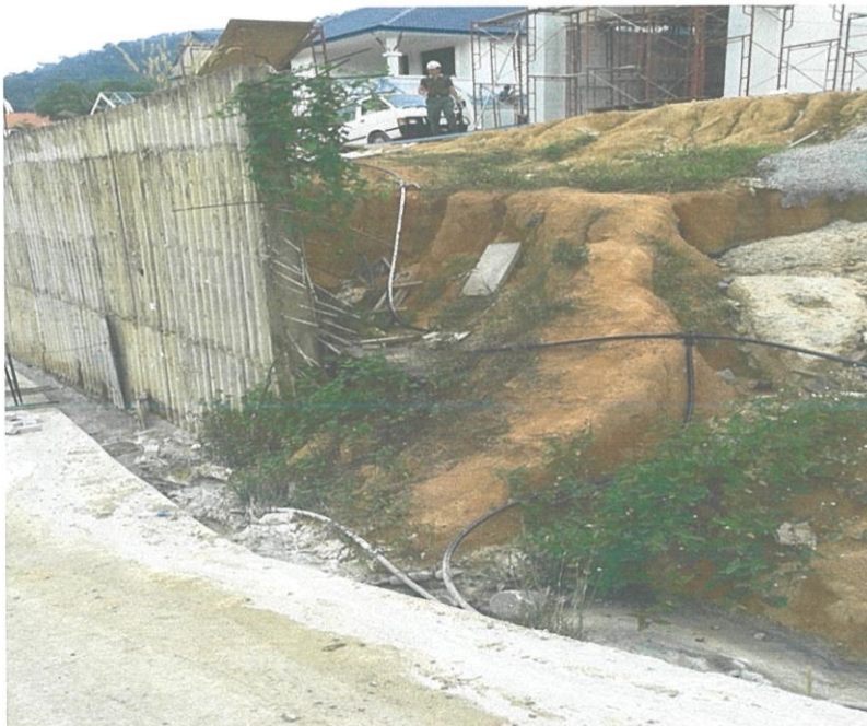
Photo 3.1: an example retaining wall to hold the high ground from falling
