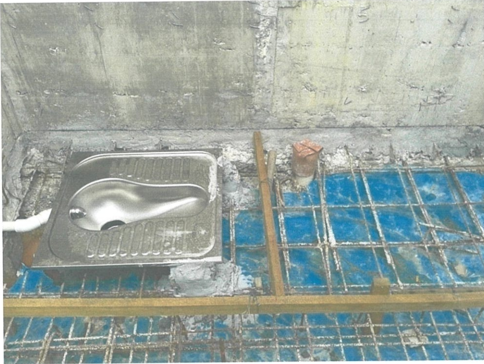
Photo 3.8 : water closet installation to every room of lockup
