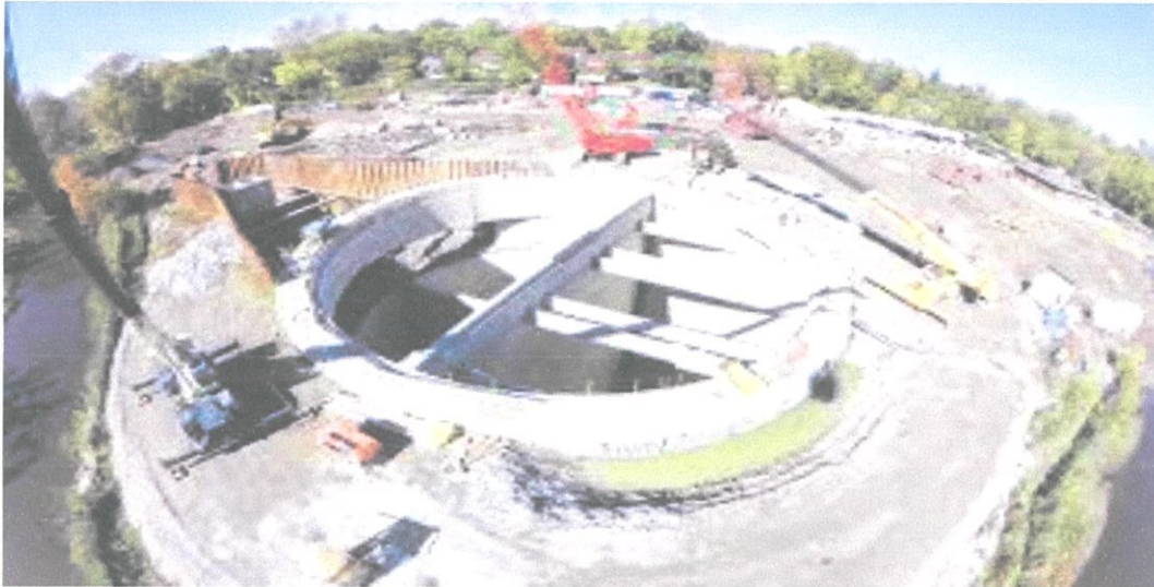
Photo 3.3 (iii): Open Caisson
