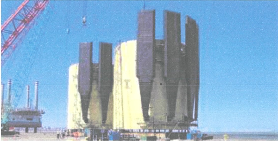
Photo 3.3 (ii): Pneumatic Caisson
