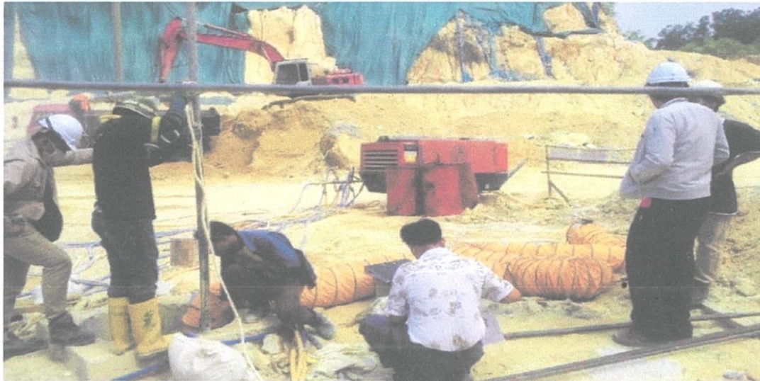
Photo 3.3 (vii): Inspection for safety ensure.
