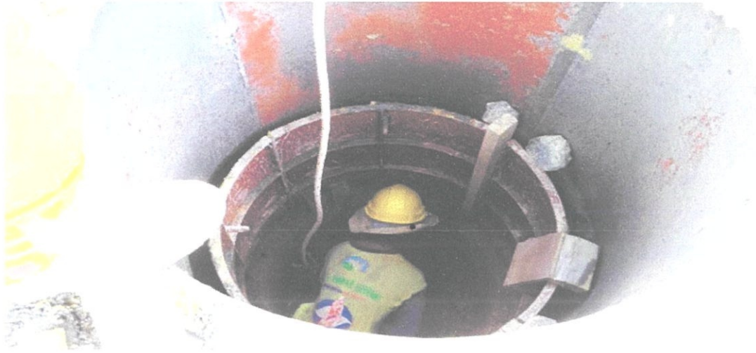
Photo 3.3 (iv): Excavated Caisson
