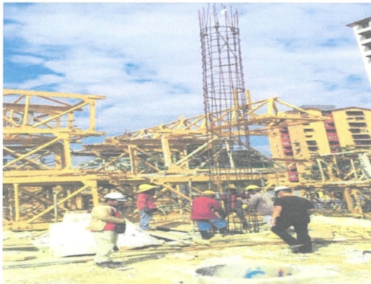
Photo 3.2: The process to erect the spiral link of Caisson.
