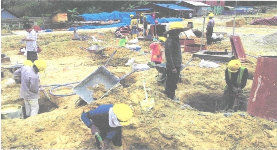
Photo 3.3 (vi): Caisson workers wear safety attire.
