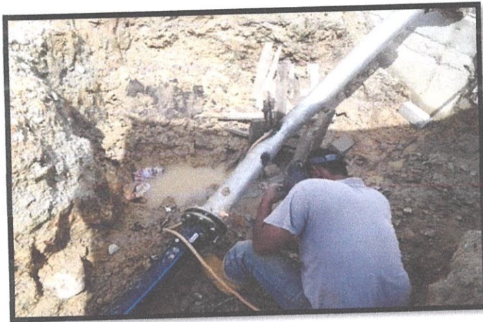
Photo 3.4 connection HDPE pipes
