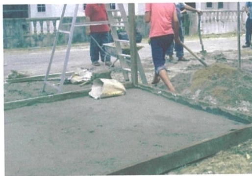
Photo 3.1 Example of cement plaster
