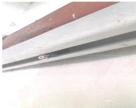
Photo 3.13: Roller stopper screwed into the Aluminum track.
