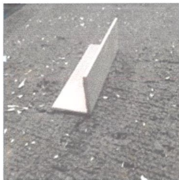
Photo 3.17: The Side fixing brackets used to support Aluminum track
