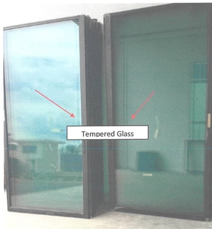
Photo 3.10: The Tempered glass used for Sliding glass door
