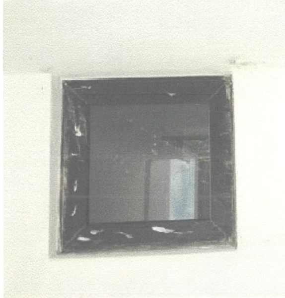
Photo 4.1: The top hung window that locate in toilet
