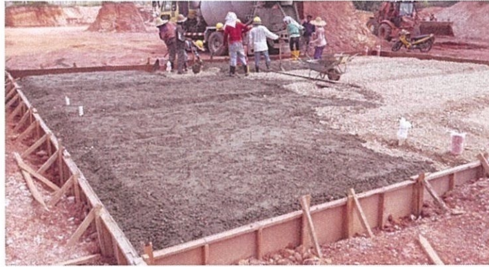
Photo 3.11: Ready Mix Concrete
