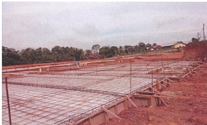
Photo 3.9: Reinforcement and DPM Layer
