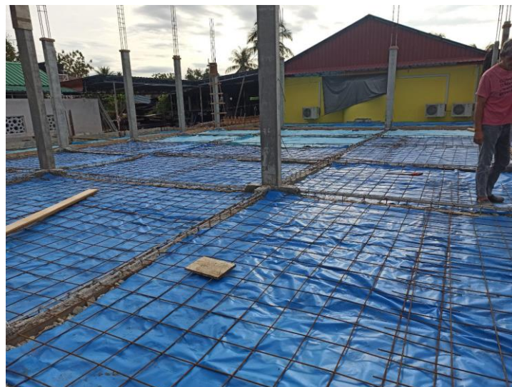
Figure 3-8 Polythene sheet and brc
