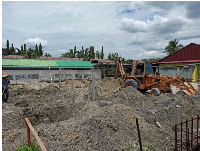
Figure 3-3 Excavation of pile cap
