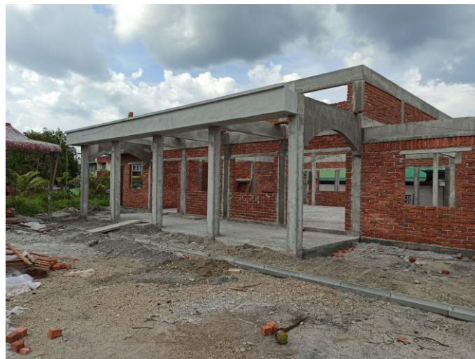
Figure 3-11 Brick works
