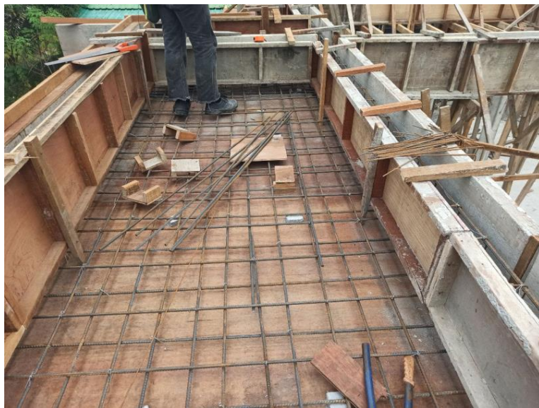
Figure 4-2 Roof Gutter Steel
