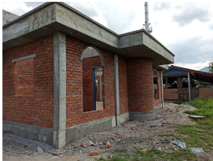
Figure 3-12 Curve Brick work
