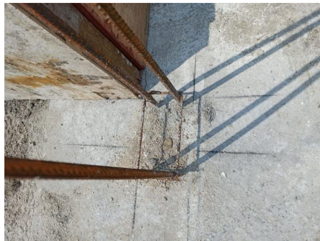
Figure 3-5 Beam marking
