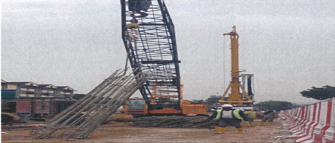
Photo 3.19 Crawler crane lifting the reinforcement cage
