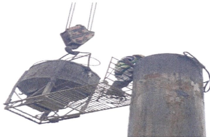
Photo 3.26 The worker was measured the final level of actual concrete
