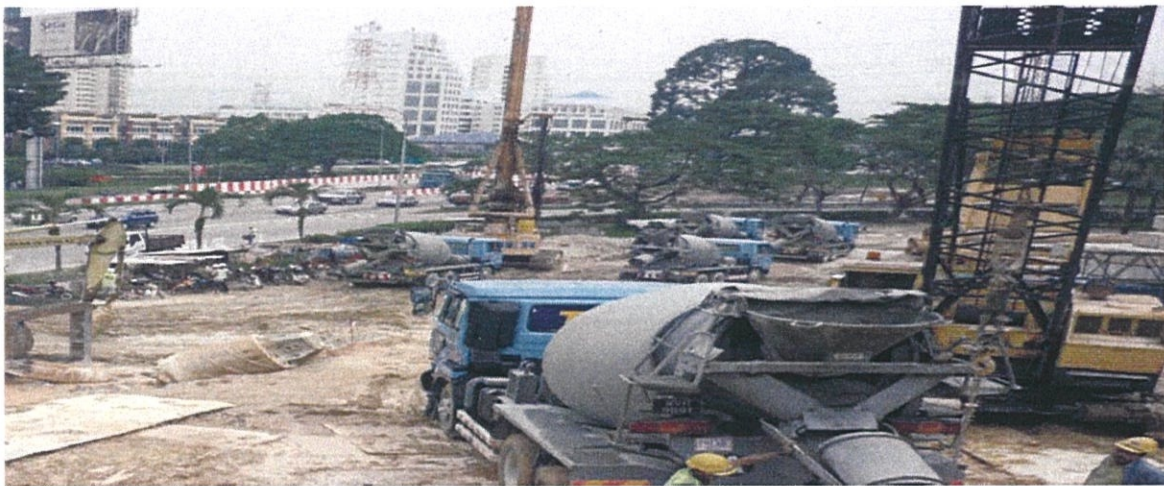
Photo 3.22 Concrete Ready-Mix Truck
