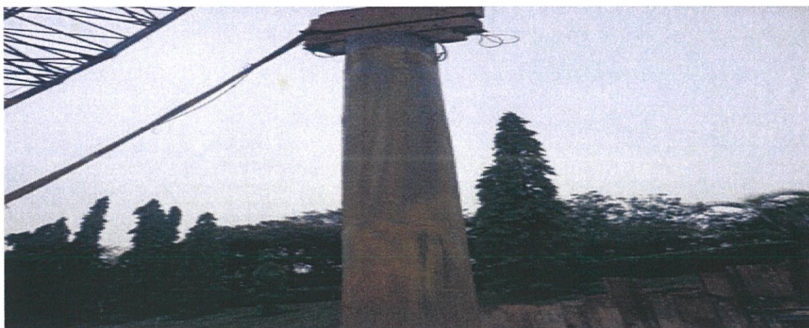
Photo 3.24 Extraction of The Temporary Casing
