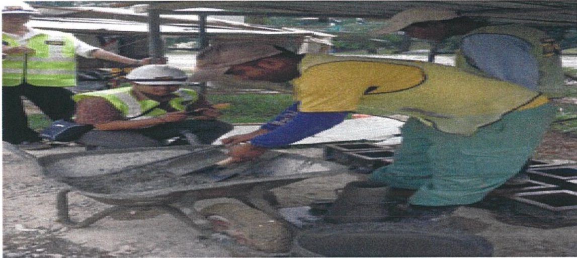
Photo 3.23 Slump Test was been carried out by the worker
