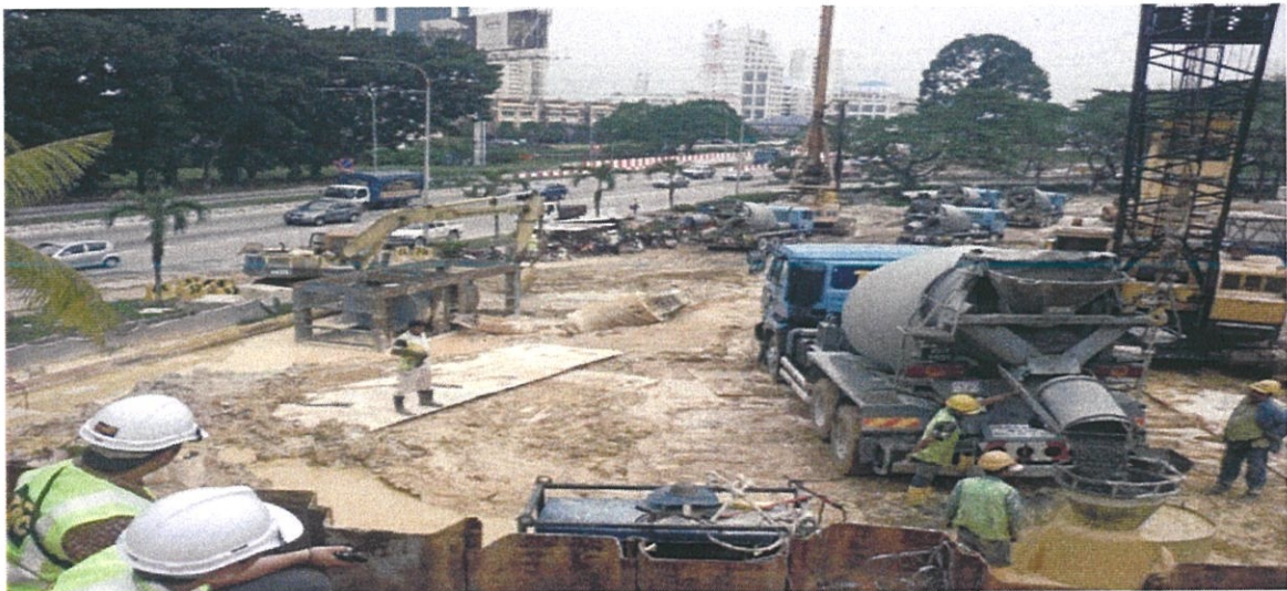
Photo 3.1 Station 3, Jalan Lapangan Terbang Subang (P66)
