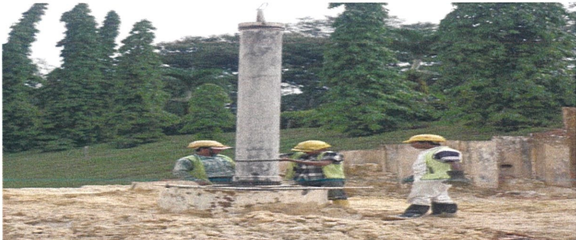
Photo 3.21 The tremie pipe was been assembled by the workers
