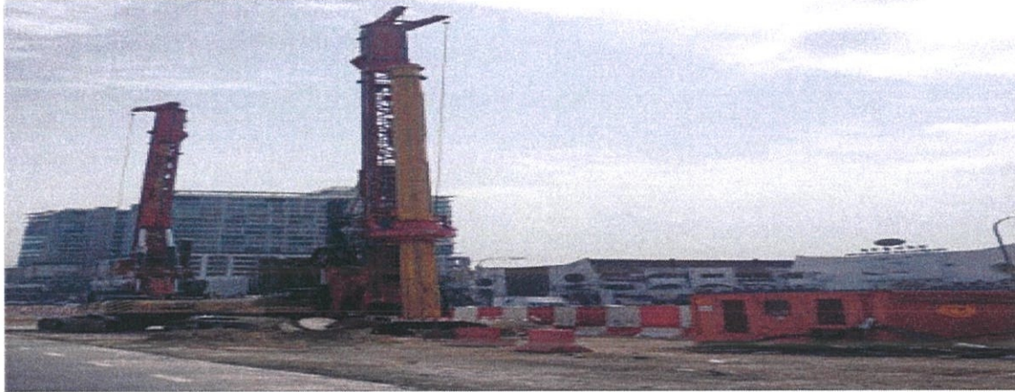
Photo 3.3 Hydraulic Boring Rig Machine
