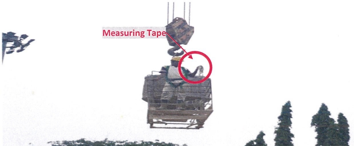
Photo 3.25 A worker was with the measuring tape to ensure the final actual level of concrete
