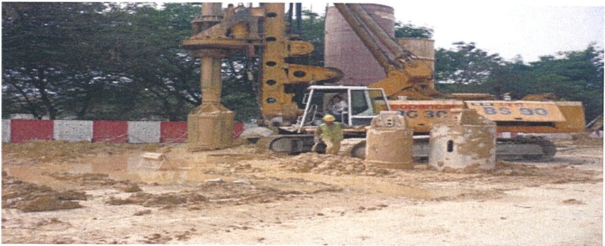
Photo 3.18 The borehole is cleaned by the cleaning bucket by lift out the drilled material
