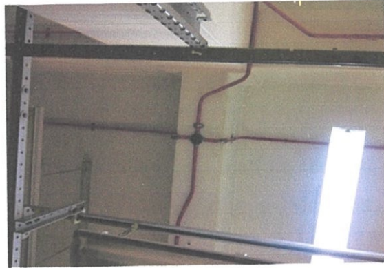
Figure 4.3: conduit has been installing
