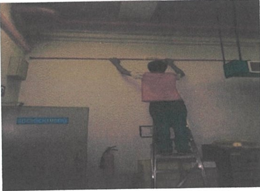
Figure 4.2: installation of conduit
