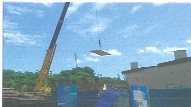
Photo 3.4 : Half slab pieces transported to the installation area by crane
