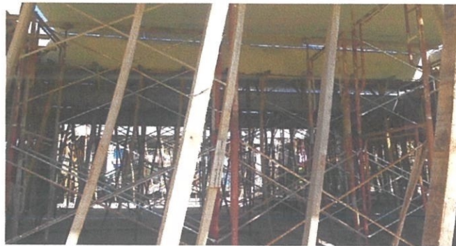
Photo 3.3 : Scaffolding for supporting installation
