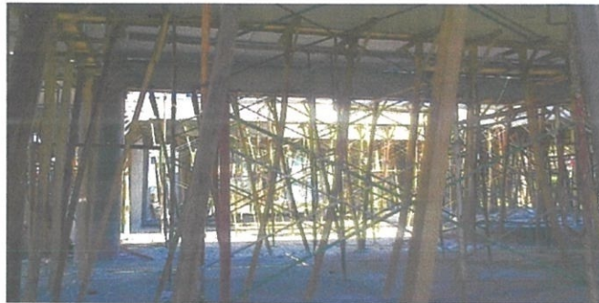
Photo 3.7 : Scaffolding were removed after concrete strength
