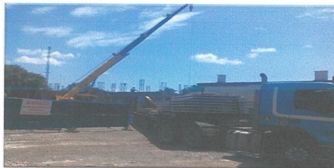
Photo 3.9 : Half slab precast concrete were install by a crane, Bukit Kepong
