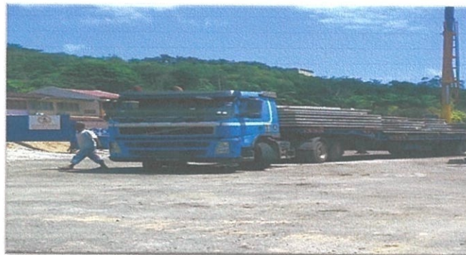
Photo 3.8 : Half slab panels were transported to site from factory using 40ft long trailer, Bukit kepong
