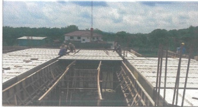
Photo 3.5 : Installation of pieces half slab
