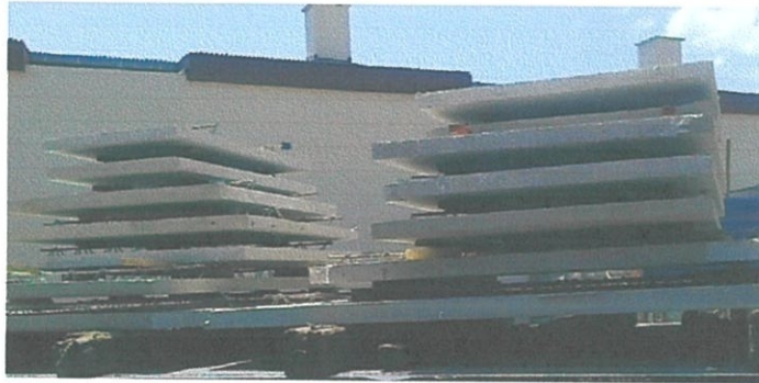
Photo 3.1 : Panels of half slab precast concrete
