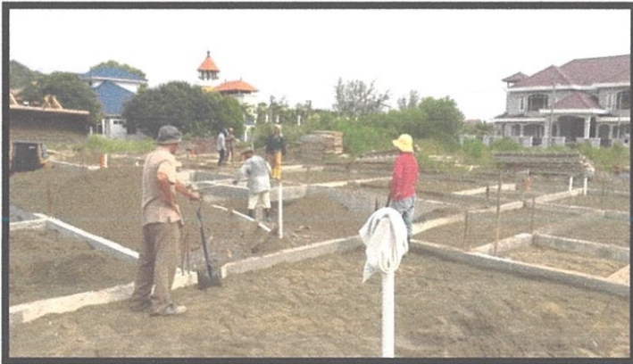
Photo 3.24 A lot of workers were smooth the soil with smoothly.
