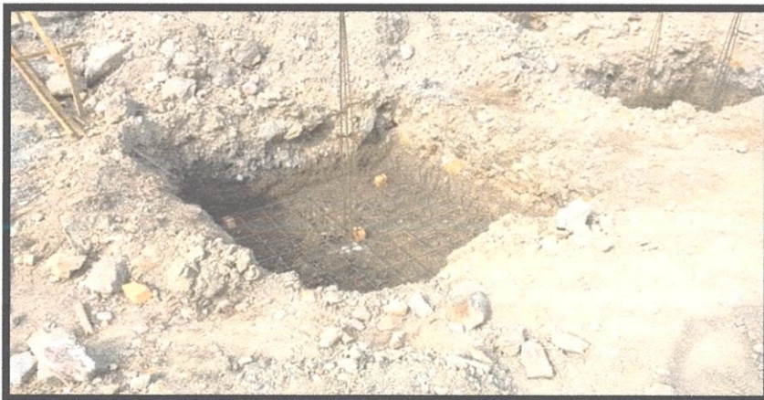
Photo 3.3 The frame of reinforcement are completed installed in the hole.
