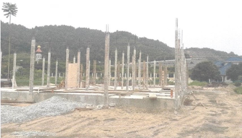
Photo 3.32 Then, the colum will install after the substructure work done.
