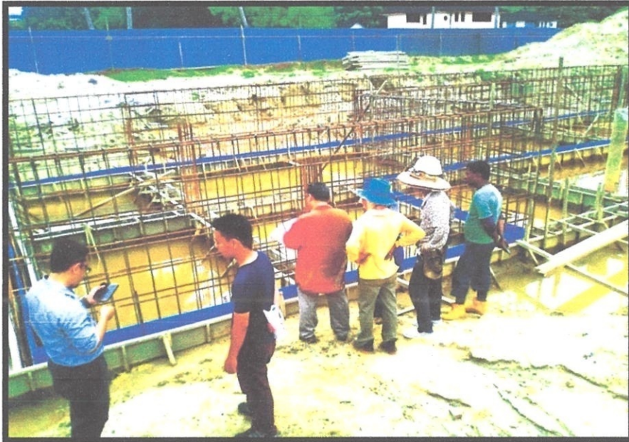
Photo 3.15 The inspection of reinforcement bars done by En Fakhurulrazi, building engineer.
