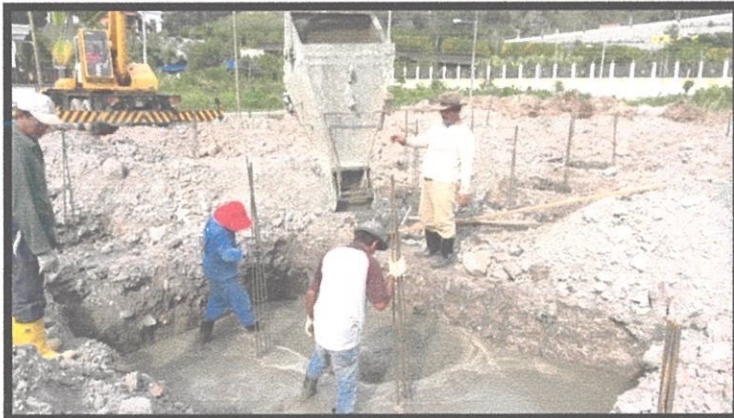
Photo 3.5 The workers are prepared to install the concrete into the hole.
