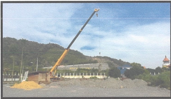
Photo 3.4 The concrete are brought by using crane
