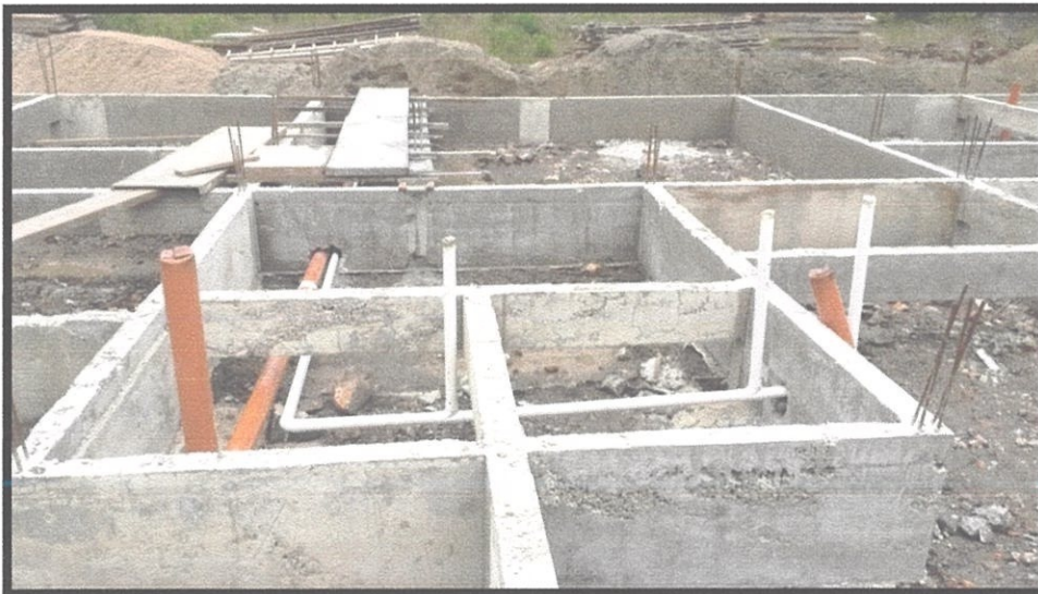
Photo 3.21 The installations of pipes
