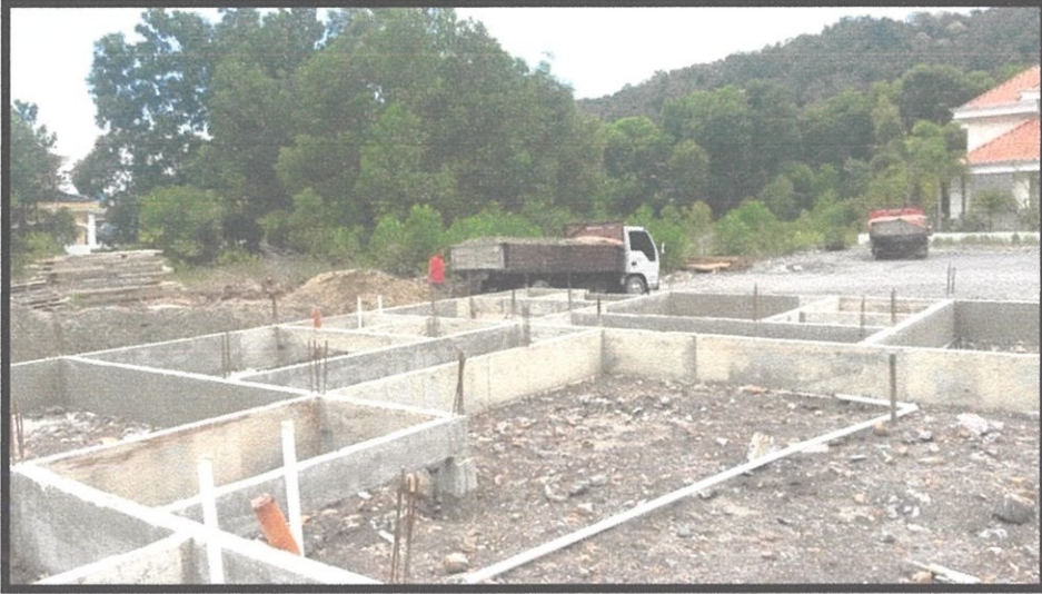
Photo 3.22 underground plumbing for the furnace utility room.
