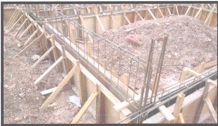
Photo 3.12 The reinforcement for groundbeam
