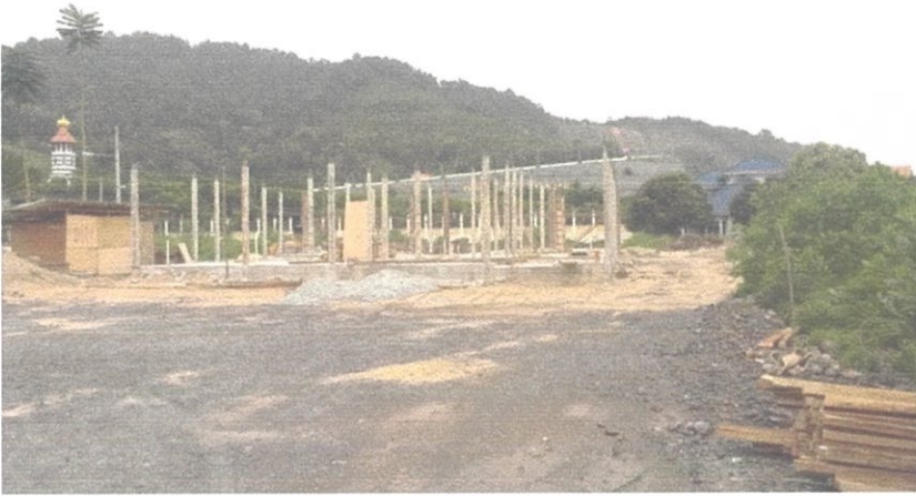
Photo 3.31 The substructure of bungalow were completely constructed.
