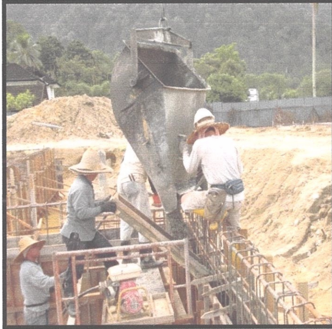
Photo 3.18 Process pouring the concrete into formwork.
