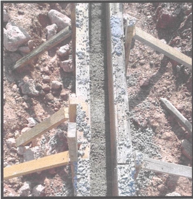
Photo 3.11 Lean concrete is poured before concreting
