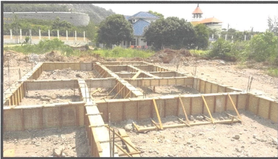
Photo 3.19 The concrete had been completely done installed
