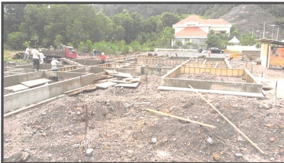
Photo 3.20 The formwork were opened and groundbeam had done
