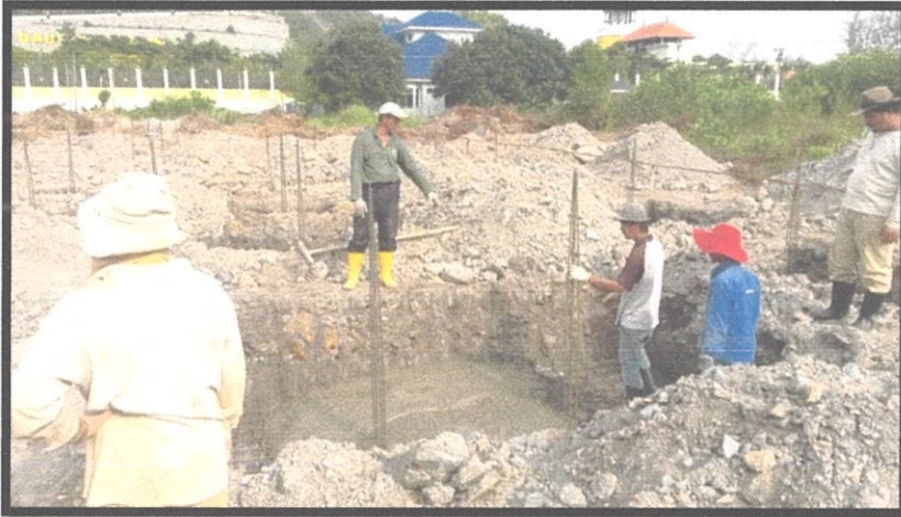
Photo 3.2 The installation of the frame reinforcement
