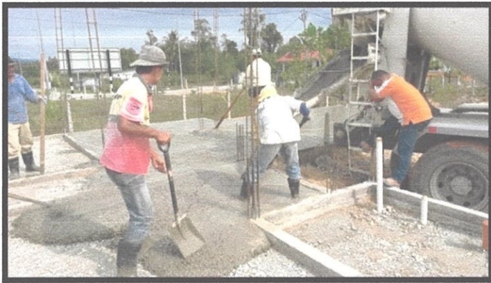
Photo 3.30 The concrete will be poured on the hardcore
