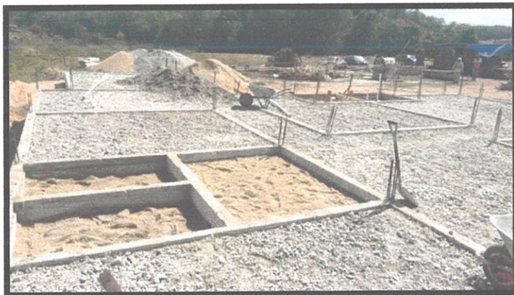
Photo 3.26 The hardcore will be compacted with hardly by a compact machine
