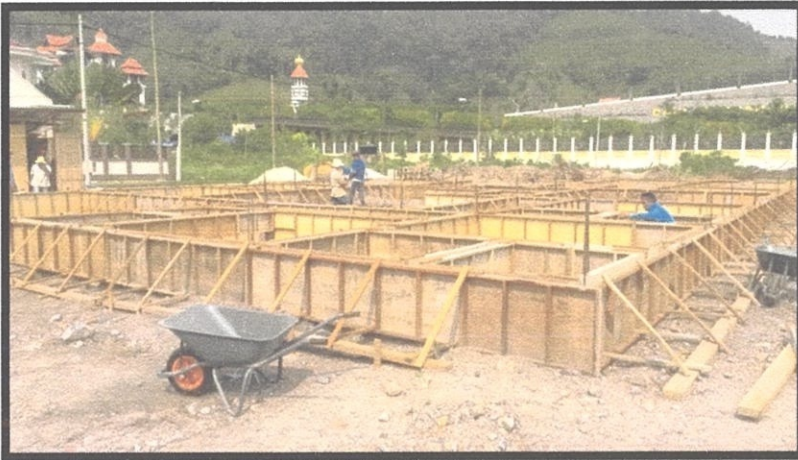
Photo 3.16 External formwork for groundbeam
