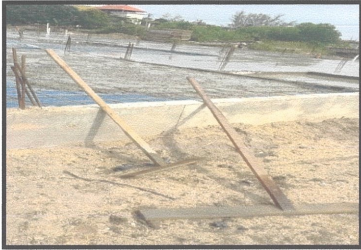
Photo 3.29 Concrete will be poured and then will be compacted
