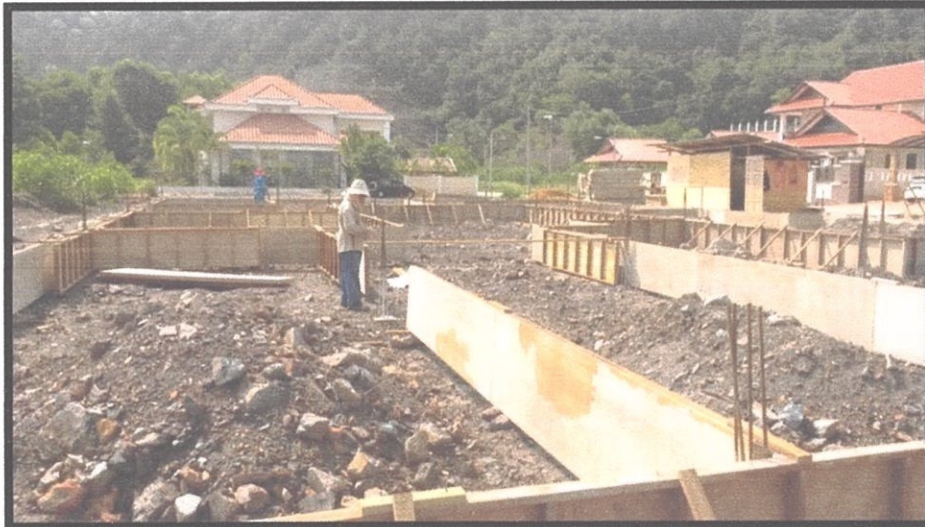
Photo 3.10 The formwork for ground beam are ready to install
