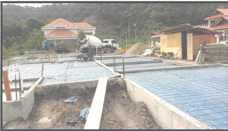
Photo 3.28 The rebars will be positioned with carefully
