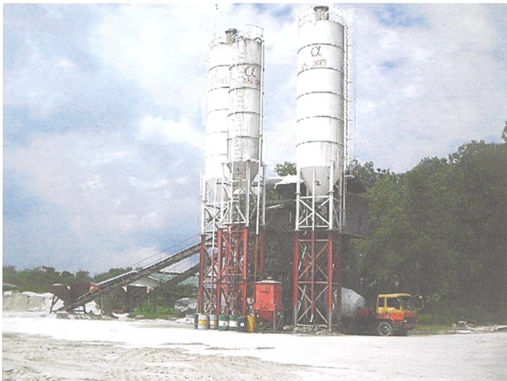
Gambar foto 4.1 Loji konkrit Alpha Concrete Sdn. Bhd.
