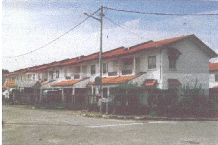
Single & Double- Storey Terrace Houses for Petronas Second Refinery Coastal Resettlement Project
