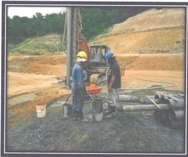
Photo 3.3.4.2 Workers pumping grout into boreholes using pipe
