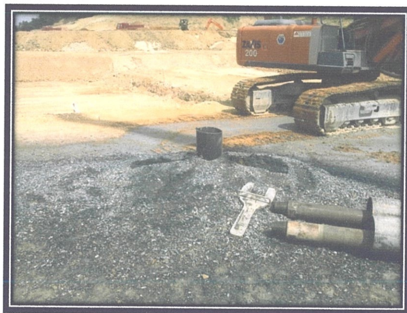
Photo 3.3.2.9 Boreholes after finishing drilling with casing
