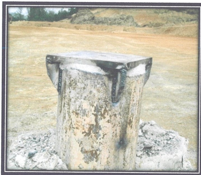
Photo 3.3.6.1.2 Metal plate welded onto footing
