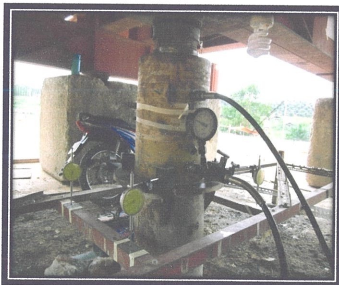
Photo 3.3.6.2.2 Hydraulics meters showing progress and change
