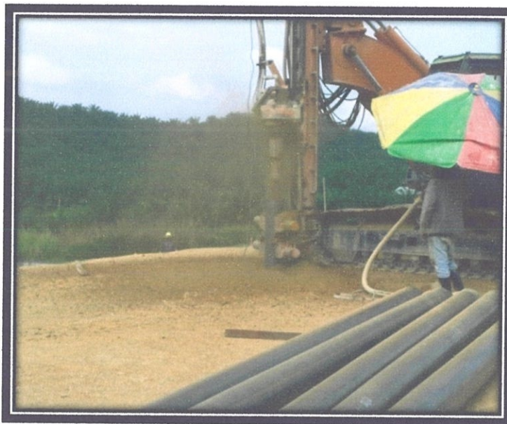
Photo 3.3.2.5 Drilling rig handled by a skilled worker
