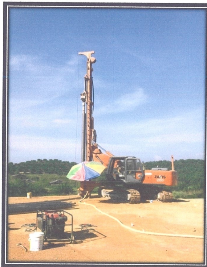
Photo 3.3.2.6 Drilling Rig on "rest mode"
