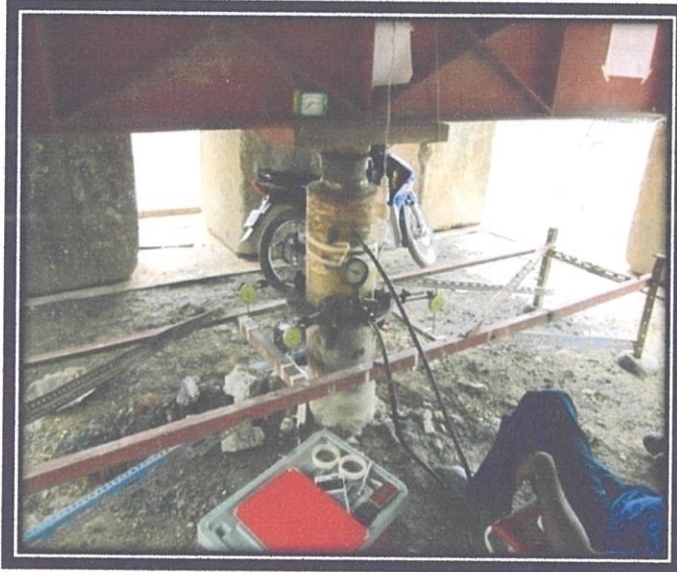
Photo 3.3.6.2.1 Hydraulic jacks being watched over for measurement
