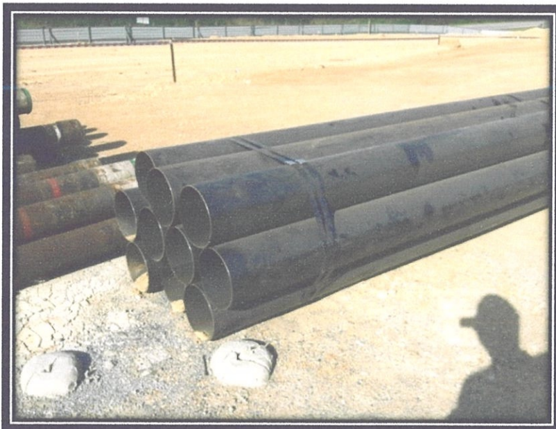
Photo 3.3.2.1 250 mm Steel Casing on site
