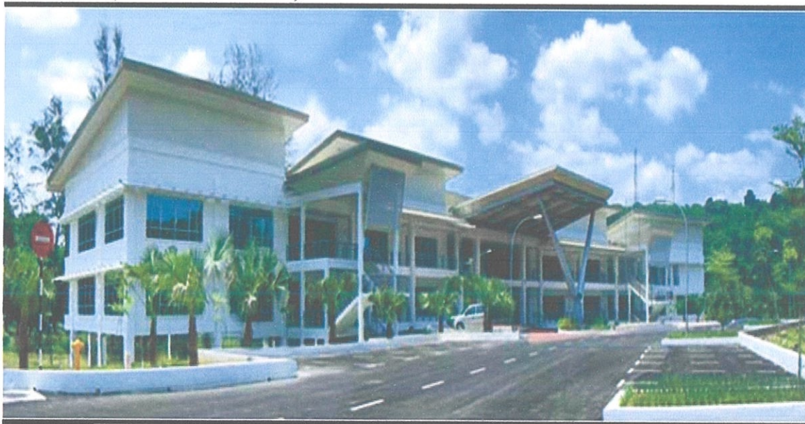
Photo 2.2.2 : This is the new JPP building used from 2011 until present time
