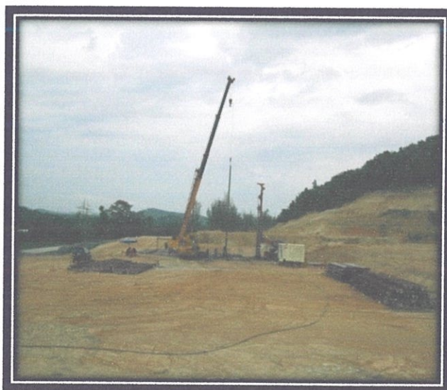
Photo 3.3.4.3 Temporary steel casing being removed from boreholes
