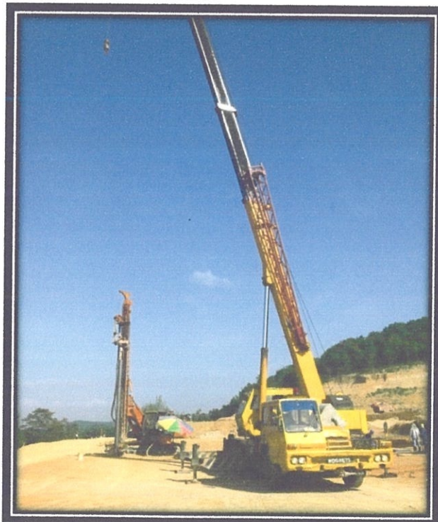
Photo 3.3.2.4 Mobile crane driven by a skilled worker
