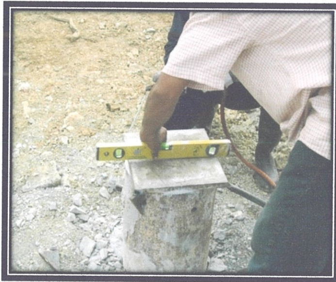
Photo 3.3.6.1.1 Worker measuring whether metal plate is stable or not
