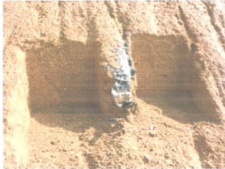
Figure 3.15 Soil nail for testing. (Draw-off tower)
