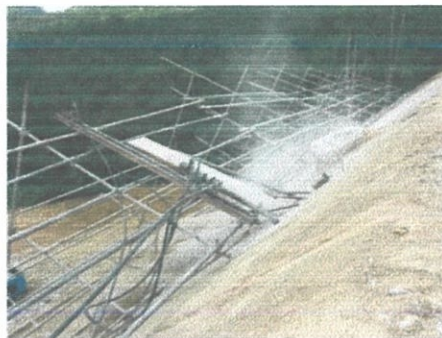
Figure 3.10 Drilling is in progress.(Draw-off tower)
