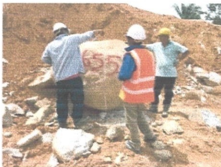
Figure 3.6 Workers are measuring the rock.(Draw-off tower)
