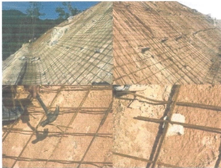
3.19 Wire mesh works.(Draw-off tower)
