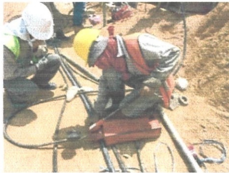
Figure 3.17 Worker jacking the stressing jack by stages. (Draw-off tower)
