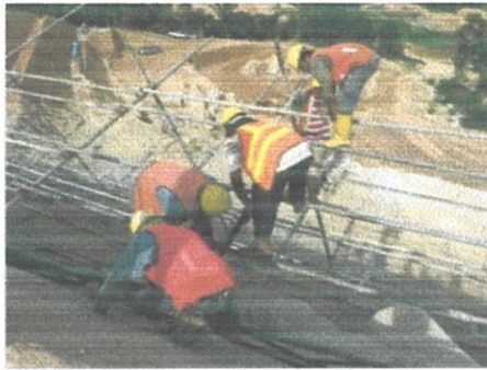
Figure 3.11 Workers are putting a soil nail components. (Draw-off tower)
