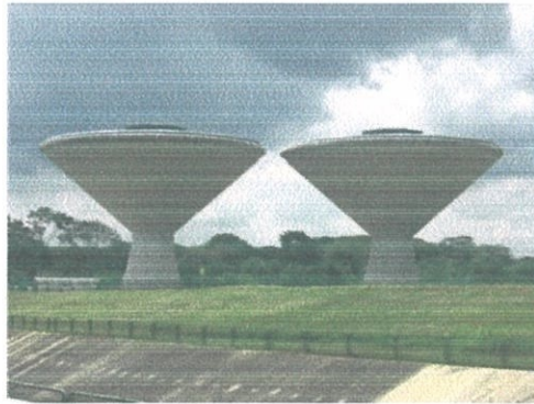
Figure 1.3 Example of Service Reservoir at Tampines Road.
