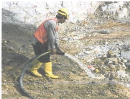
3.29 Workers remove unwanted materials using water. (Valve House)
