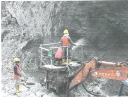
Figure 3.34 workers splaying the shotcrete (Valve House)
