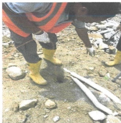
Figure 3.26 Worker installing the explosive material.(Draw-off tunnel)
