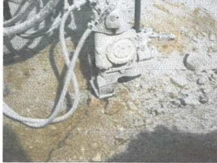
Figure 3.23 Drill machine.(Draw-off tunnel)
