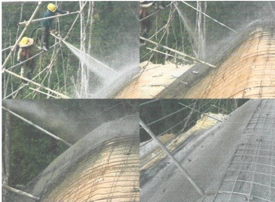
Figure 3.21 Guniting works.(Draw-off tower)
