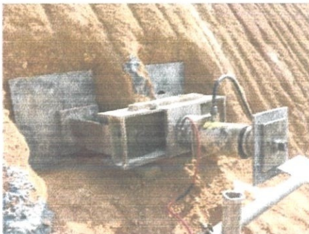
Figure 3.16 Soil nail pull-out test equipment. (Draw-off tower)
