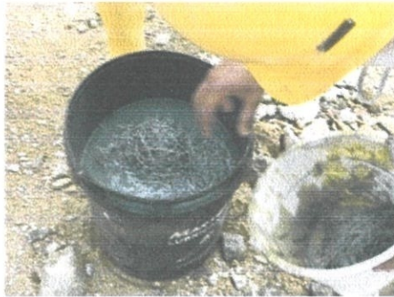
Figure 3.32 Separated steel fiber. (Valve House)
