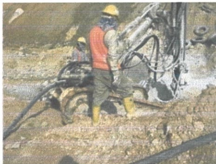
Figure 3.22 Workers are checking the equipment. (Draw-off tunnel)
