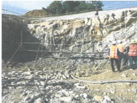
Figure 3.30 Temporary staging for safety. (Valve House)
