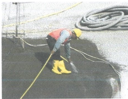
Figure 3.35 curing process. (Valve House)
