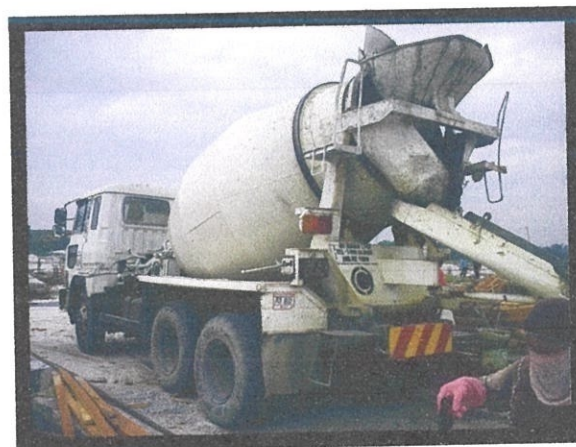
Photo 3.17: The concrete mixer lorry
