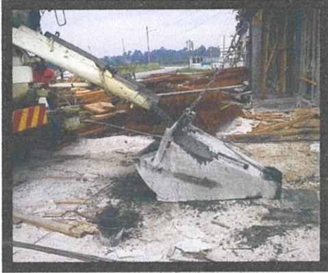
Photo 3.18: The bucket of concrete
