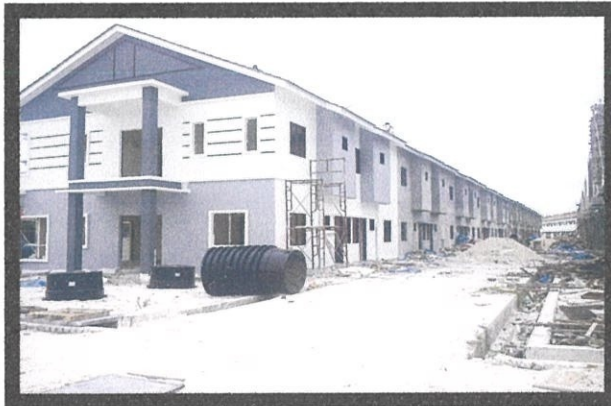
Photo 3.1: The view of double storey terrace house from the rear
