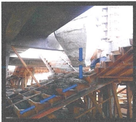
Photo 3.20: The workers poured the concrete to the forms.
