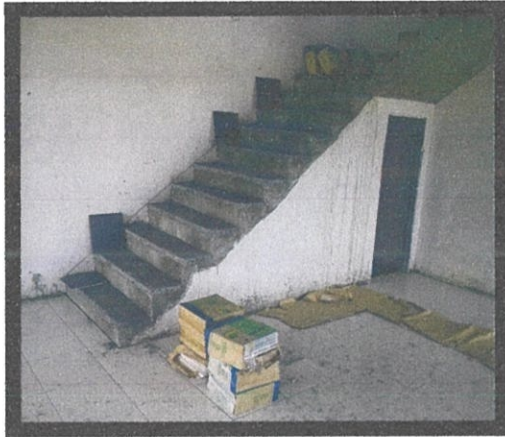
Photo 3.28: The staircase surface that was marked
