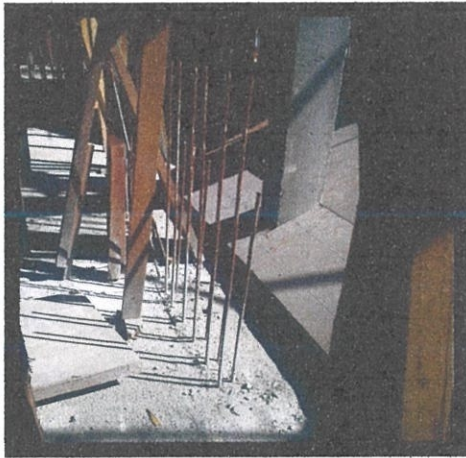
Photo 3.10: The bonding bars at the ground floor.
