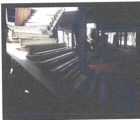
Photo 3.26: The staircase after dismantle the riser
