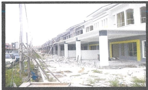
Photo 3.2: The view of double storey terrace house from the front
