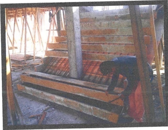
Photo 3.12: The workers installing the timber panels
