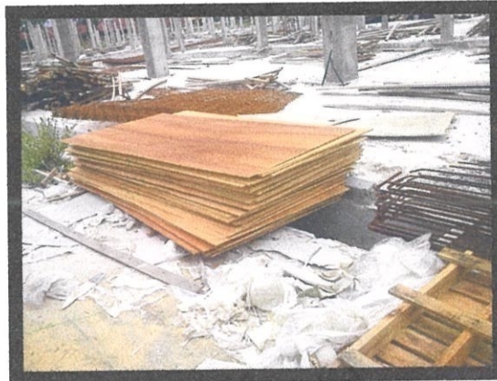
Photo 3.4: The low grade timber board which will be cut and shaped
