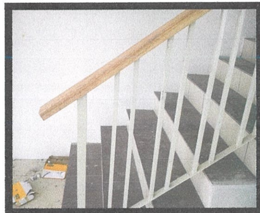
Photo 3.31: The handrail and baluster were installed to the stair
