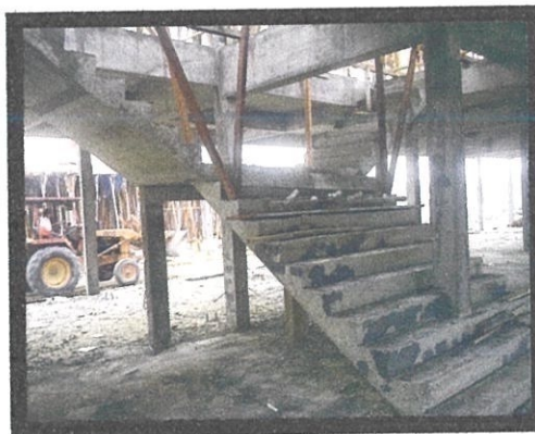
Photo 3.27: The staircase after remove the riser boards
