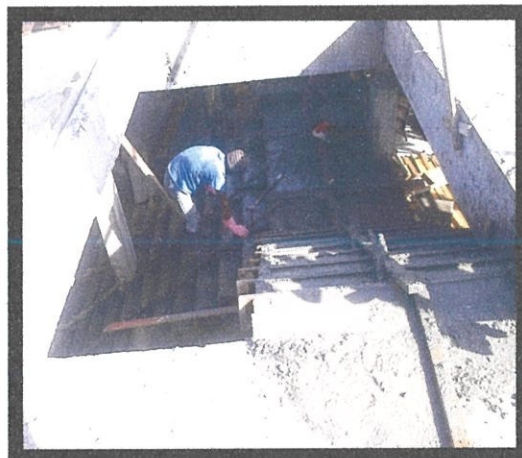
Photo 3.24: The workers flatten the surface with steel trowel.
