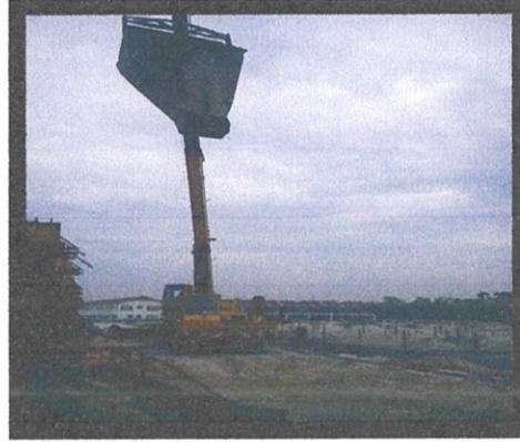
Photo 3.19: The mobile crane carrying the bucket
