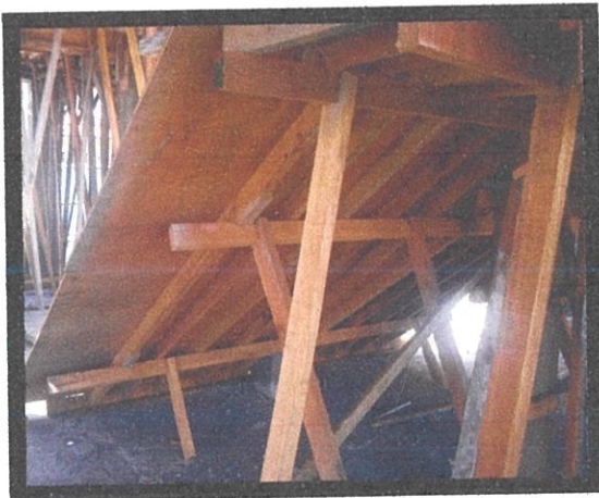
Photo 3.7: The wooden bracing which supports the forms
