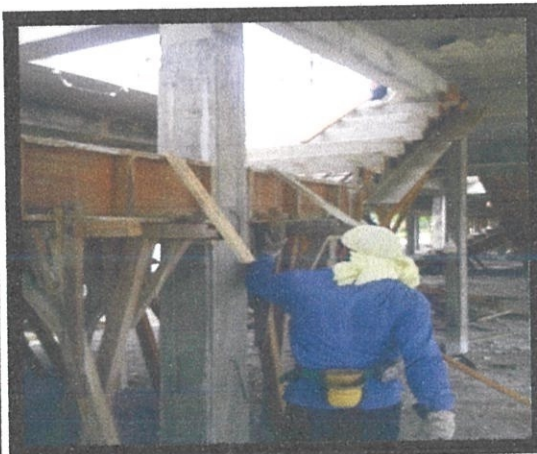
Photo 3.8: The worker installed the wooden braces
