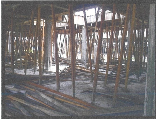
Photo 3.3: The view of the area which the stairs will be constructed
