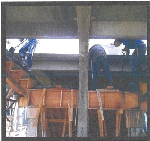
Photo 3.23: The workers transport the excess concrete to upper panels
