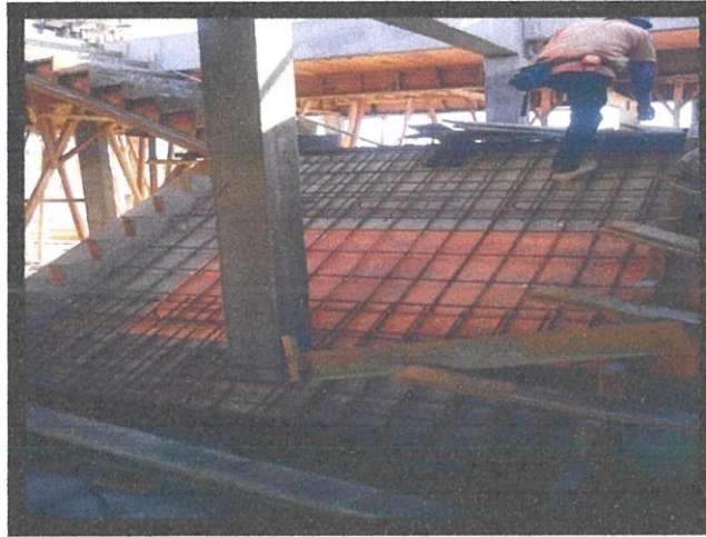
Photo 3.9: The worker installed the reinforcement bar.
