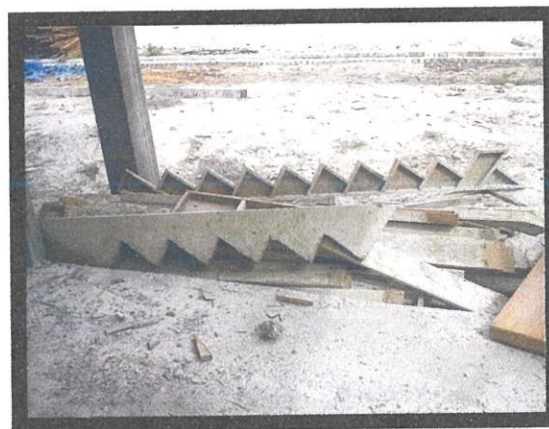
Photo 3.5: The side forms which cut from the timber boards
