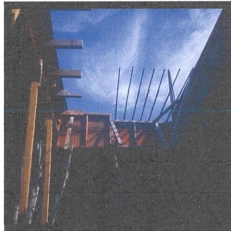
Photo 3.11: The bonding bars at the first floor
