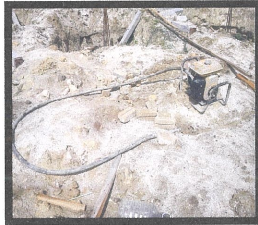
Photo 3.22: The concrete vibrator
