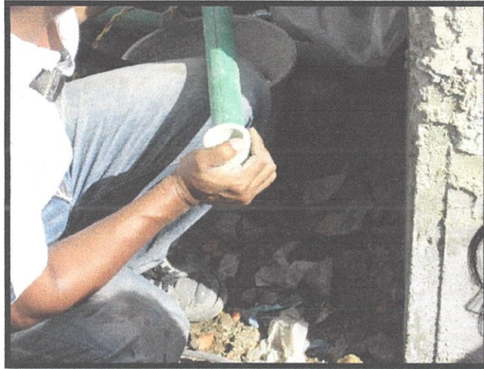
Photo 3.7 The pipe is fitting together until the depth is reached
