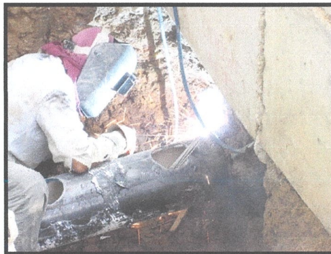
Photo 3.12 Welding the collar to jointing that pipe
