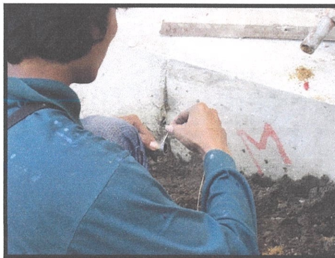
Photo 3.18 Use the thread to be placed in the thread line
