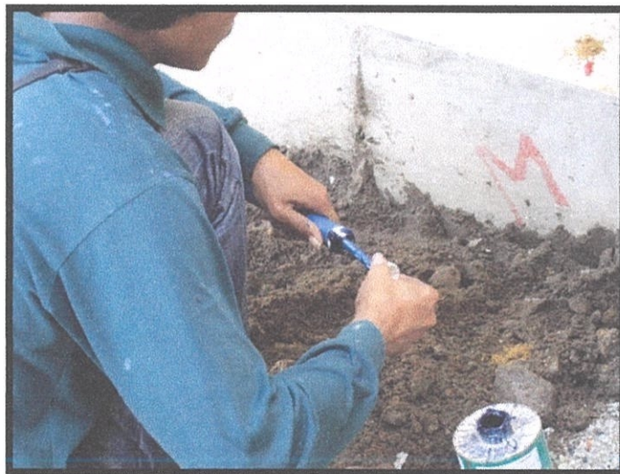
Photo 3.20 use the upvc glue again to stiking that white tape
