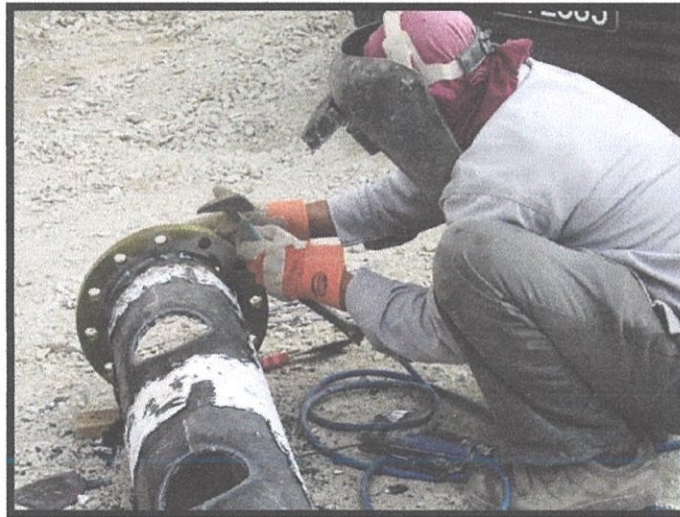
Photo 3.10 Remove the excess sheet metal
