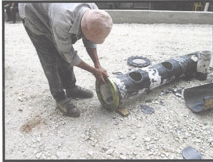
Photo 3.8 The flange must be positioned
