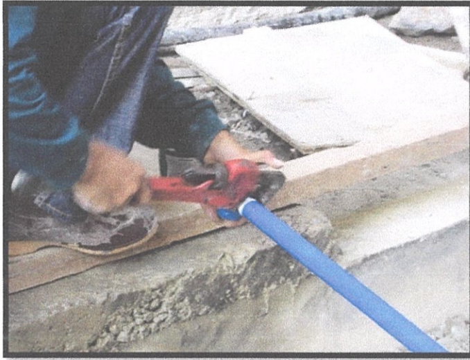
Photo 3.21 Use pipe wrench to strengthen and tighten the pipe installation
