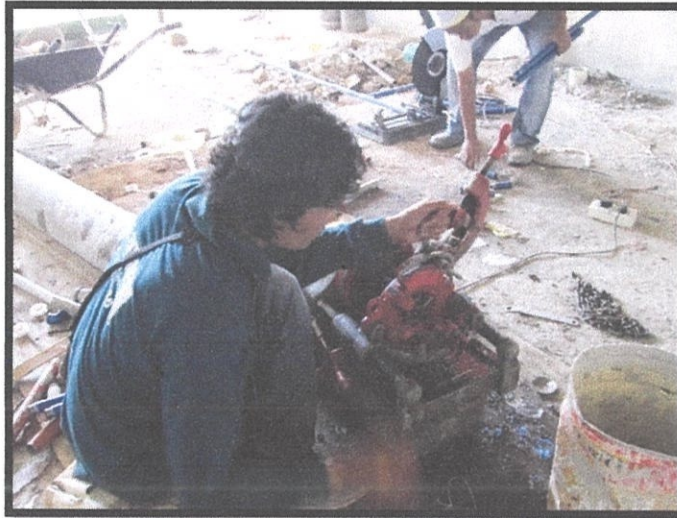
Photo 3.17 Threading Process
