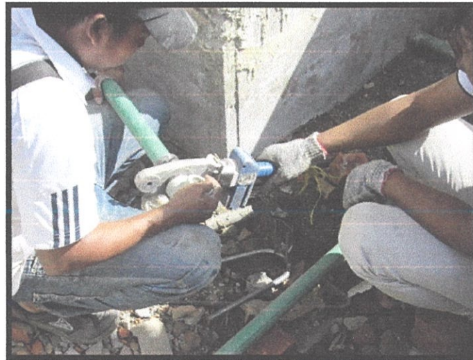
Photo 3.6 The pipe is pushed and fitting into the welding adaptors
