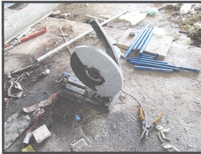
Photo 3.14 The poly steel pipe has been cut
