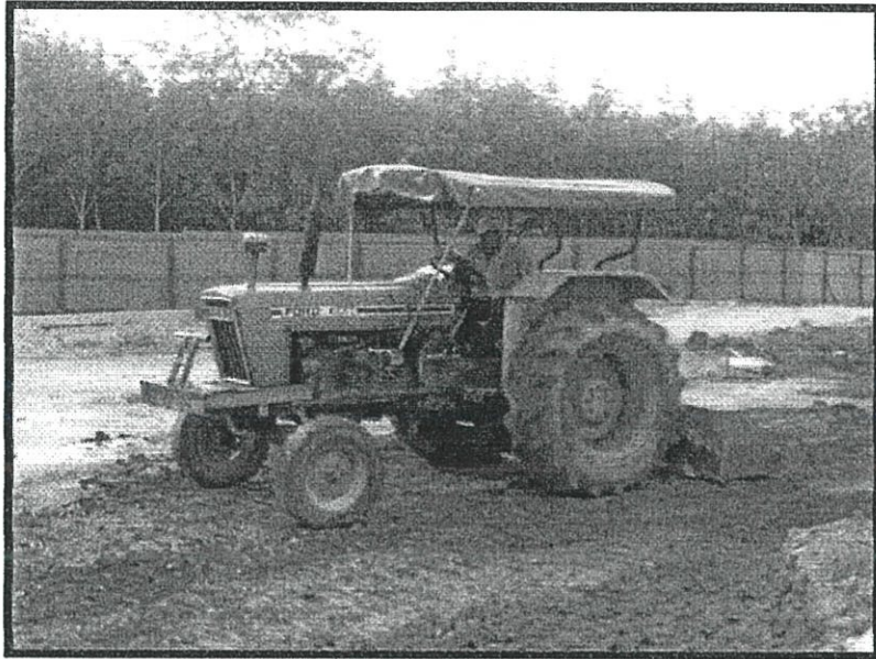
Gambar Foto 4.3 :Backpusher
