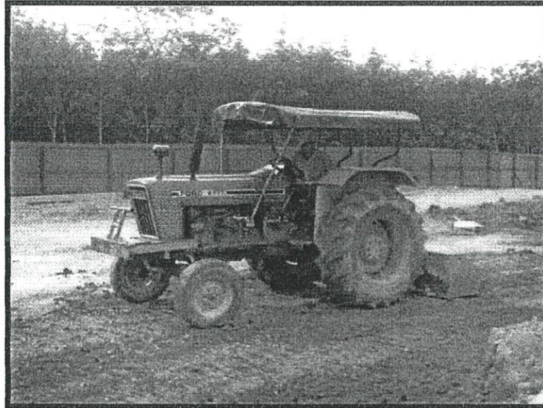
Gambar Foto 3.4: Backpusher
