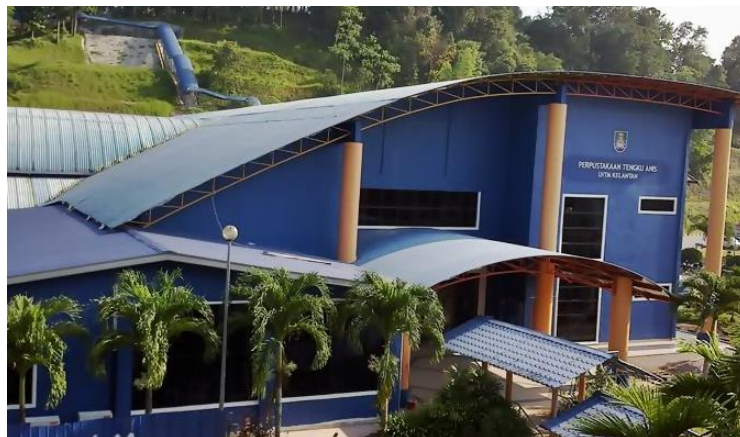
Figure 1: The PTA building
