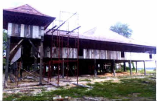
VISIT TO ALICE FORT (UNDER MAINTENANCE) 22 AUGUST 2014
