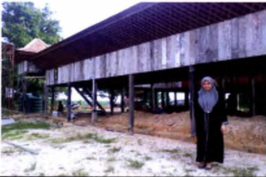
VISIT TO ALICE FORT (UNDER MAINTENANCE) 22 AUGUST 2014
