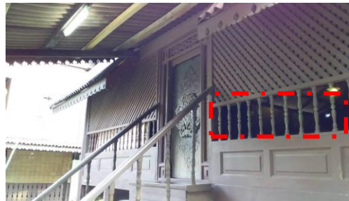
Figure 1.2: Rumah Negeri Sembilan with decorative elements (Source: Awaludin, 2019)
