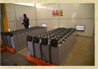
The 28.13kW standalone solar PV system is supplying electricity to 28 households of Iban community in the Rumah Panjang. The system was commissioned on November 2021 and designed to operate with 60% of the consumption supplied by battery and 40% by the solar PV.
