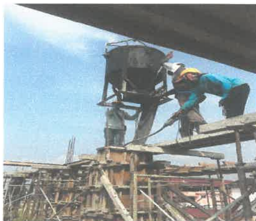
Figure 8.8: Observing the workers pouring concrete to beam structure.
