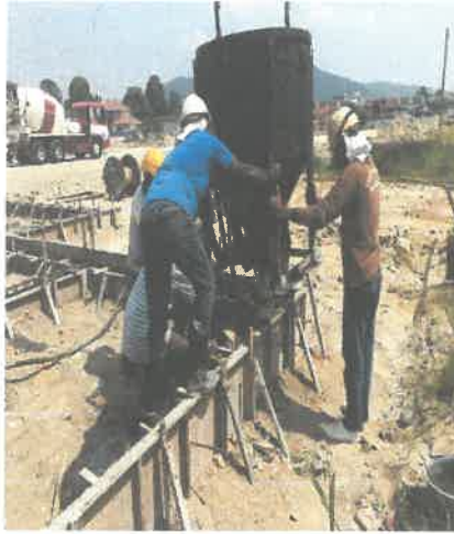
Figure 8.3: Supervising workers pouring concrete.
