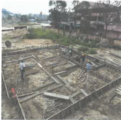
Figure 8.4: Supervising the workers constructing formwork.
