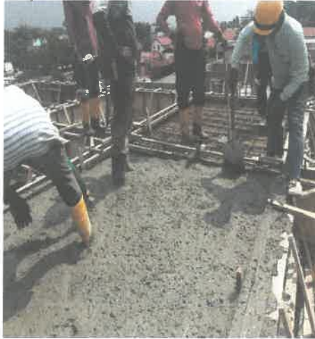
Figure 8.6: Supervising the workers pouring concrete to slab structure.
