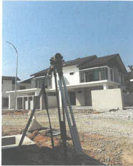
Figure 8.1: Using dumpy level for levelling
