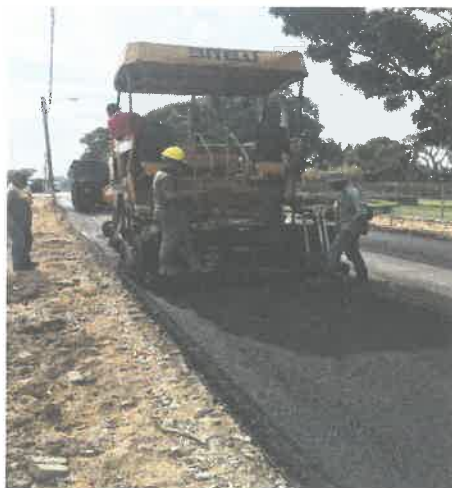
Figure 8.5: Supervising subcontractor on roadwork construction.
