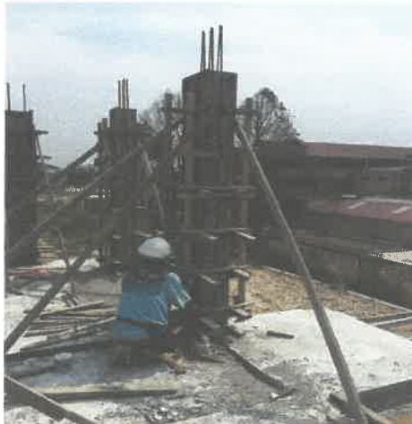
Figure 8.7: Observing the workers aligning the formwork of column.
